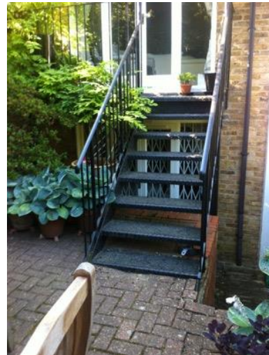
Existing access to balcony and steps to lower ground floor.
