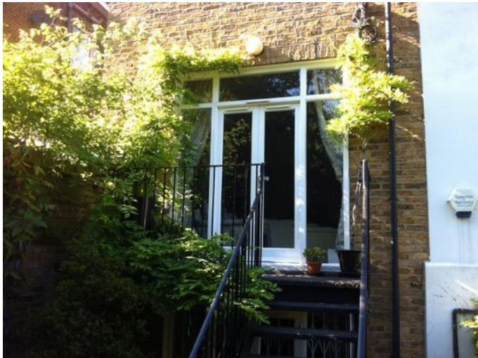
Existing balcony at ground floor level and steps towards the garden
