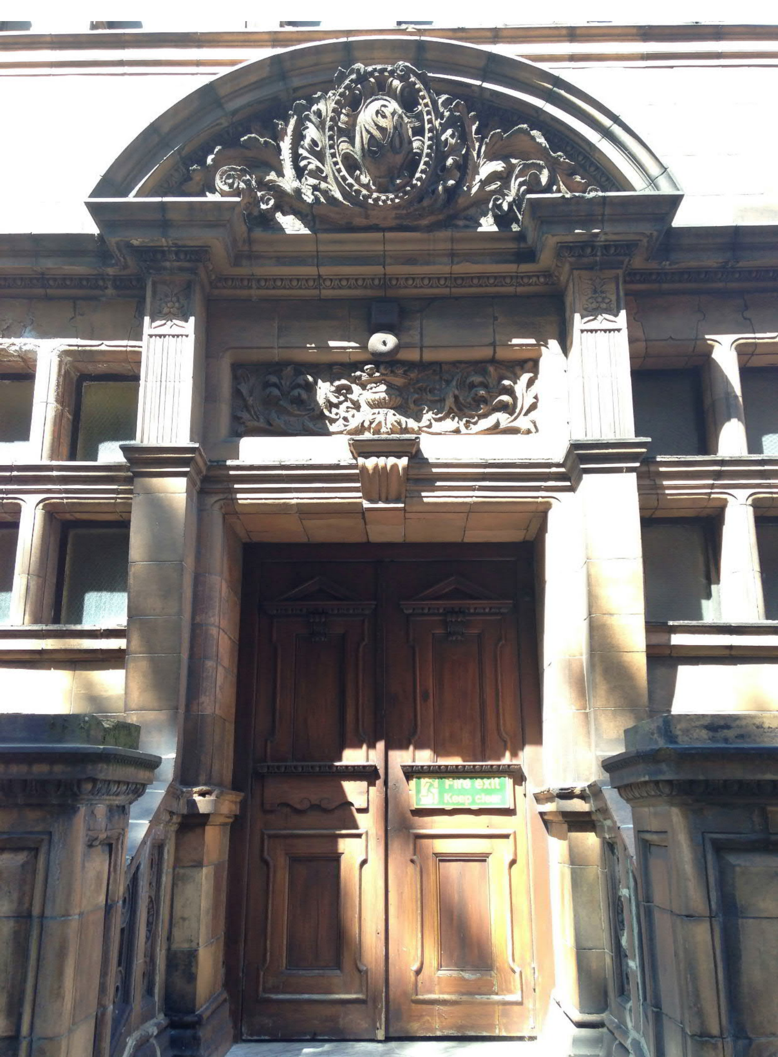
Existing Sign 10 - Fire Exit Keep Clear.JPG
