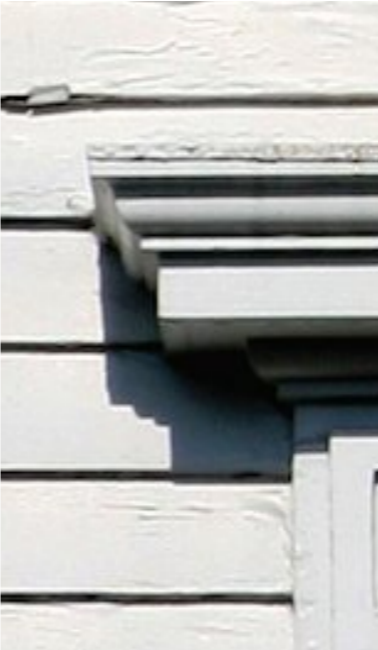
3 Restore original Stone Front Elevation Windows.
