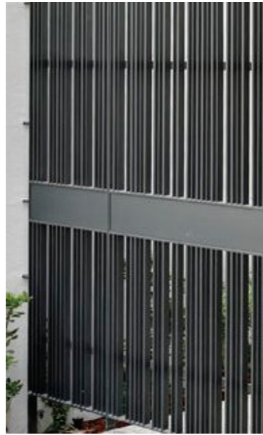
H Garden Gates to be designed in a similar style to the Main Entrance Gates. The slender vertical rails provide a light, delicate style to respect the existing building. They also have a neutral style to extenuate the historical merit of the existing buildings.
