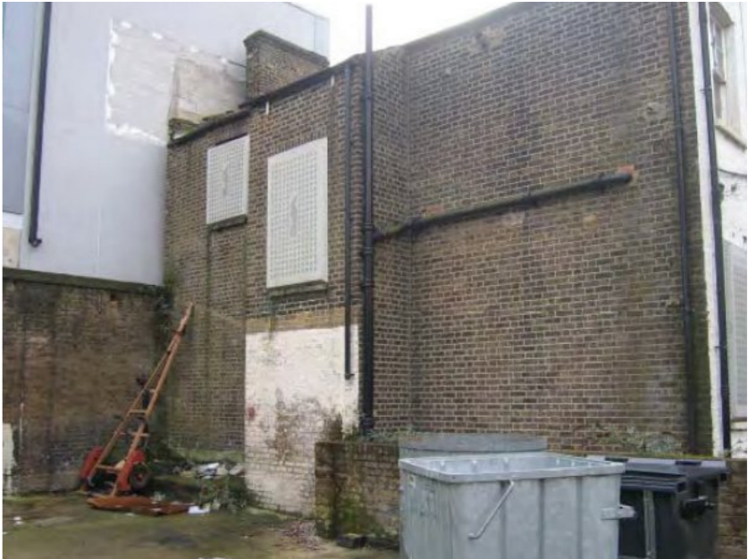
2 Existing view of the house at the rear elevation
