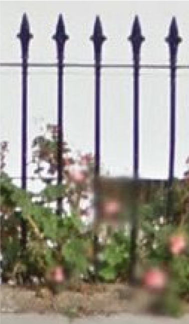
8 Restore and Repair Existing Railings.
