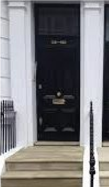
4 Restore and Repair Existing York Stone Steps. Entrance Door to be painted Black and to receive new Bronze Ironmongery.
