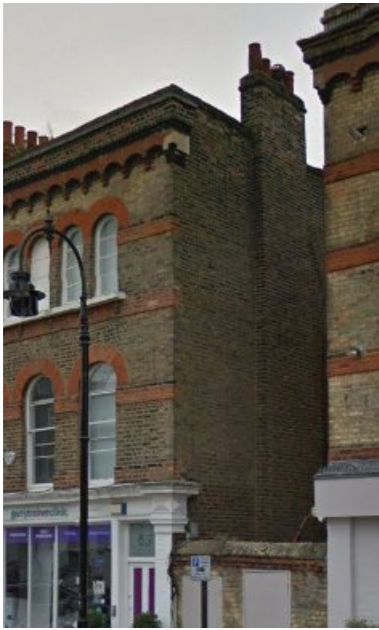
A Chimney Stack to be expressed on the Gable Facade - as per the example above at 65 Princess Street adjacent to the site.
