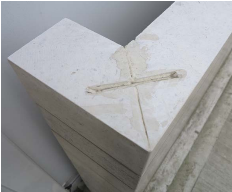
All corners mitred to avoid unwanted exposed joints
