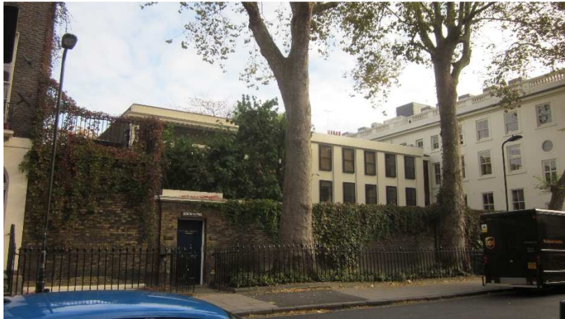
View of 29a from Montague Street
