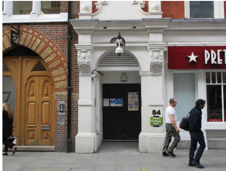
Figure 1 - Front elevation existing louvre
