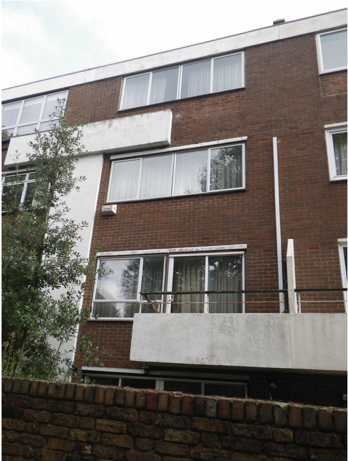
IMAGE 06: View of rear elevation
