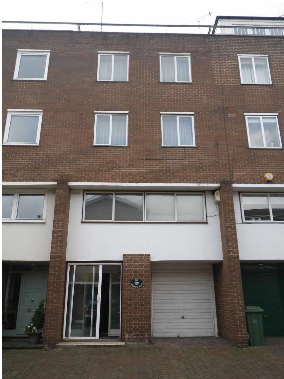
IMAGE 01: Front elevation, view of no. 20 from Meadowbank
