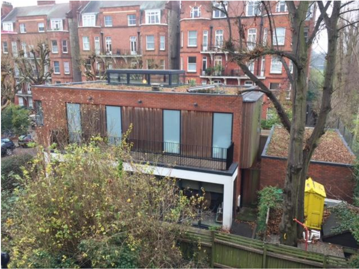
Photo 3: Side (east) elevation when viewed from second floor flat in Clevedon Mansions
