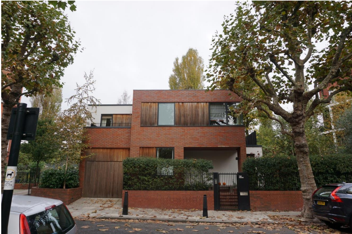
Photo 1: Front (south) elevation of existing house
