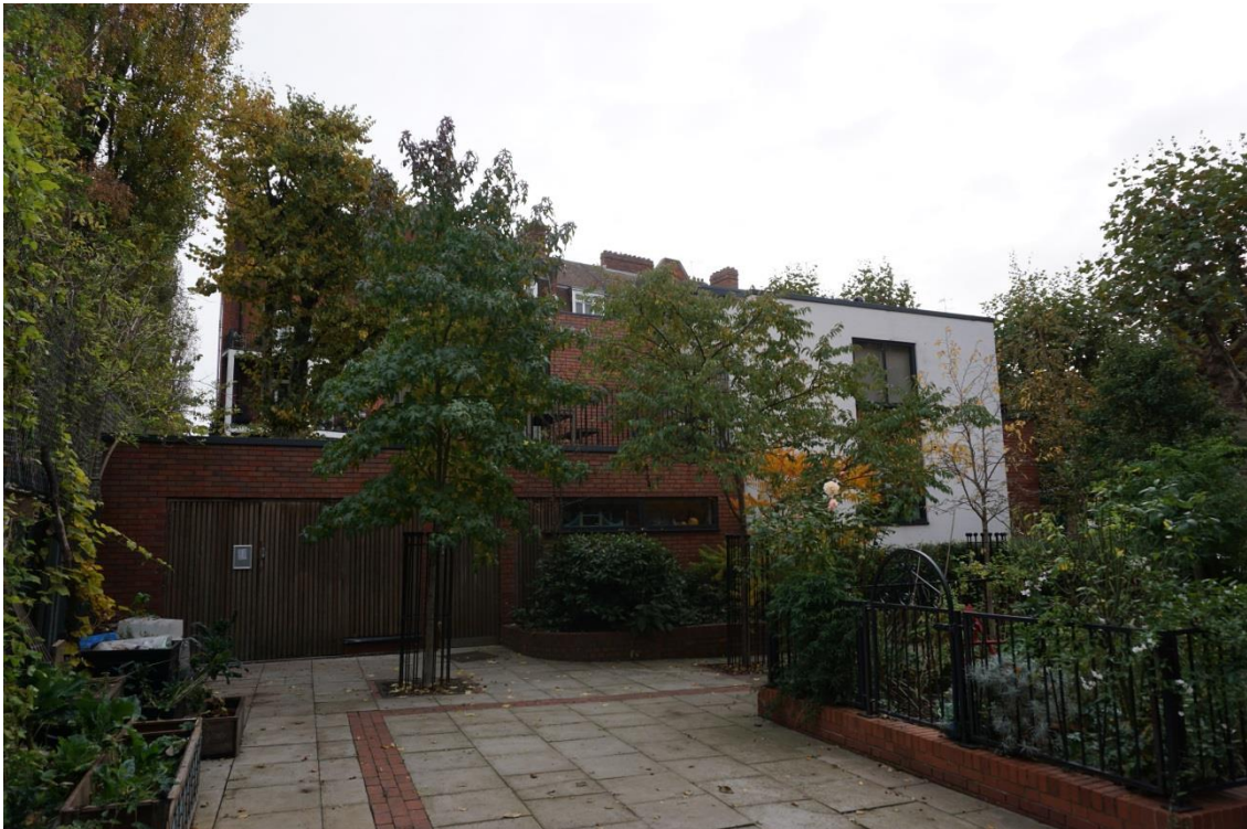
Photo 10: Western elevation as viewed when approaching from walkway leading to Hampstead Heath
