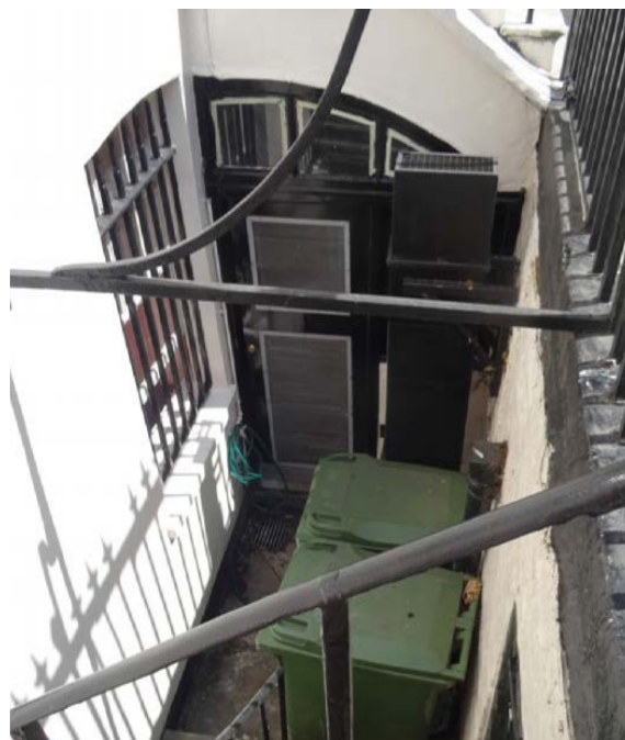
Existing Basement Access from Street
