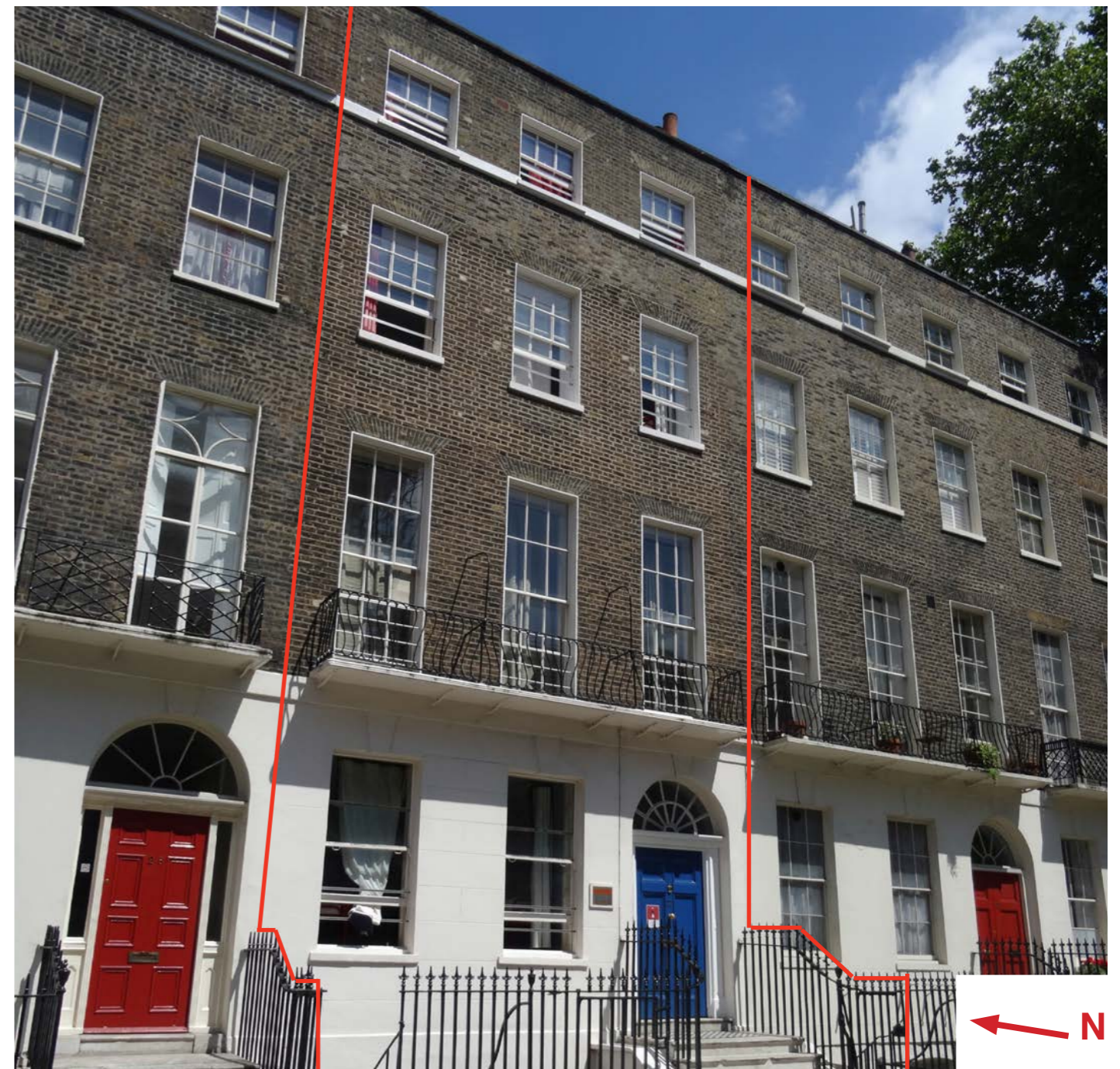
Montague Street, View of terrace with No. 27 outlined in red.
