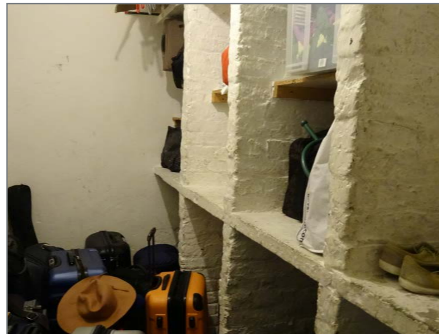
Existing Wine Cellar
