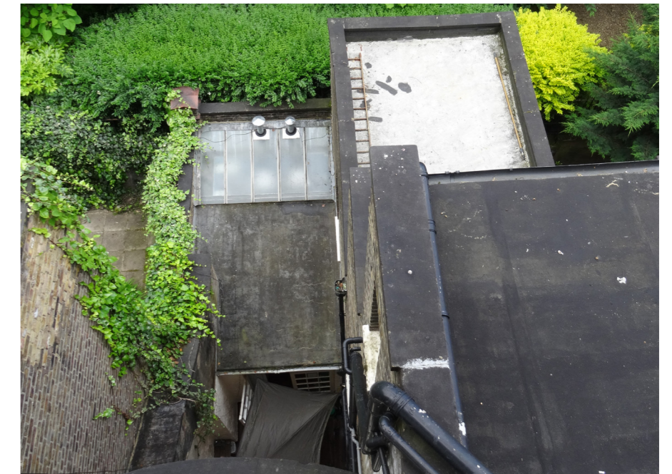
Outlook from Rear window of Second floor over Rear Extension
