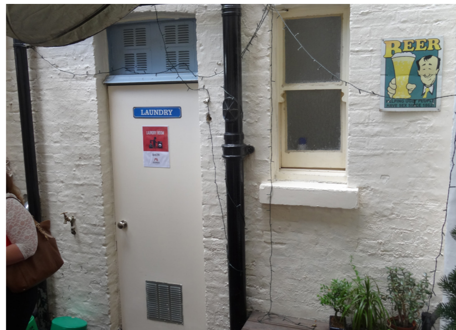
Existing Basement Courtyard looking into Laundry Room Entrance
