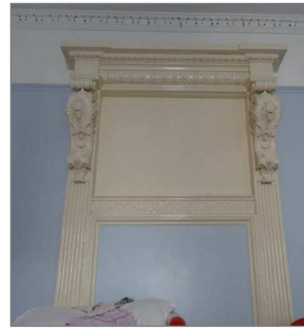
Sealed Decorative Doorway at 1st Floor
