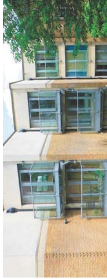
8 Stepped vernacular to the rear of Burghley Court; cantilevered balconies with glazed double doors
