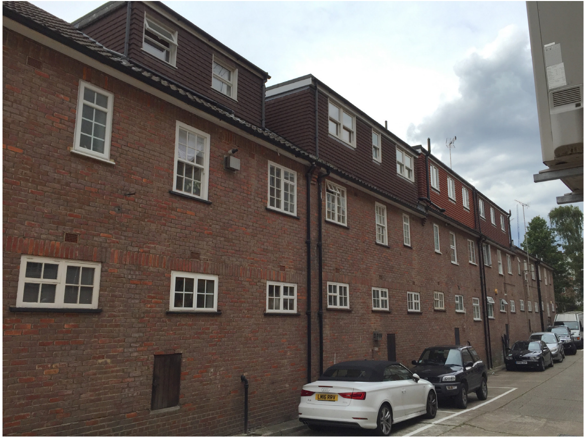
looking north along rear of 16-26 Fairfax Place facing onto private service road
