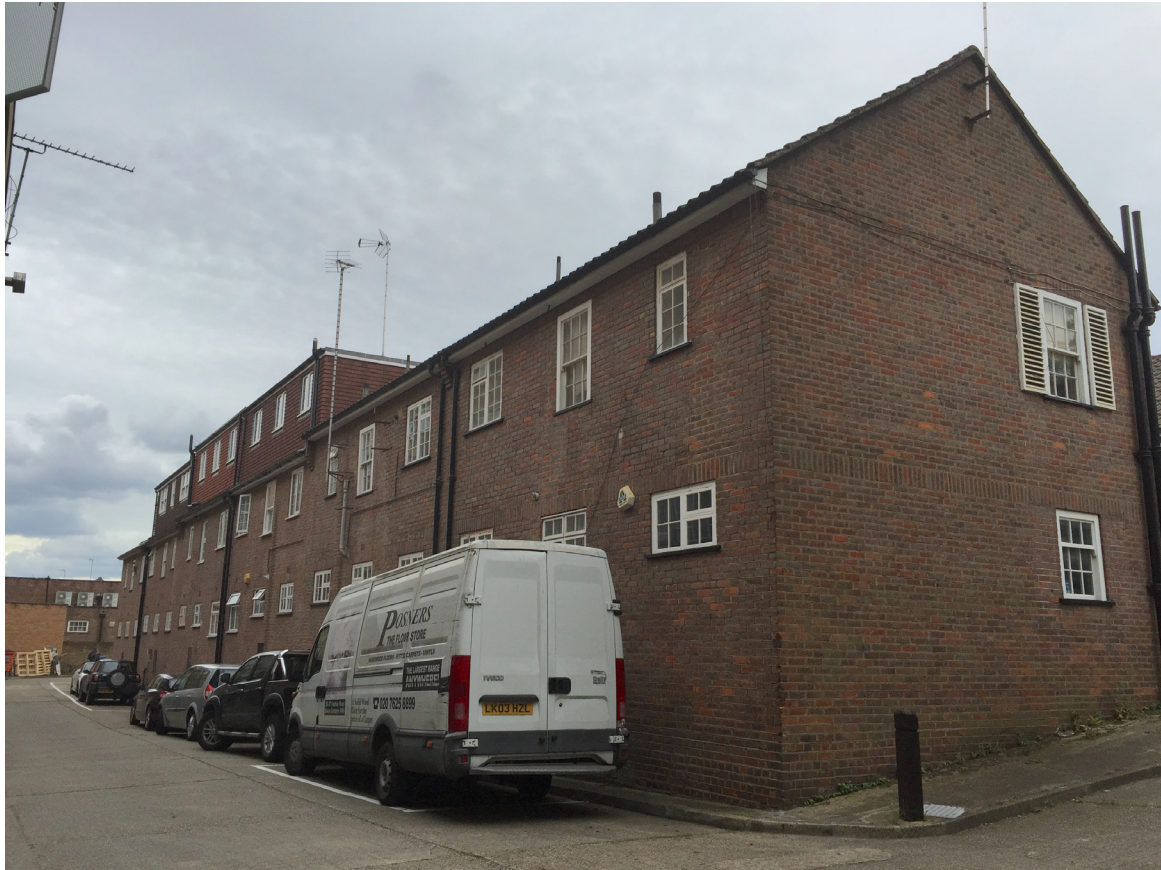
private service road to rear of 16-26 Fairfax Place looking south
