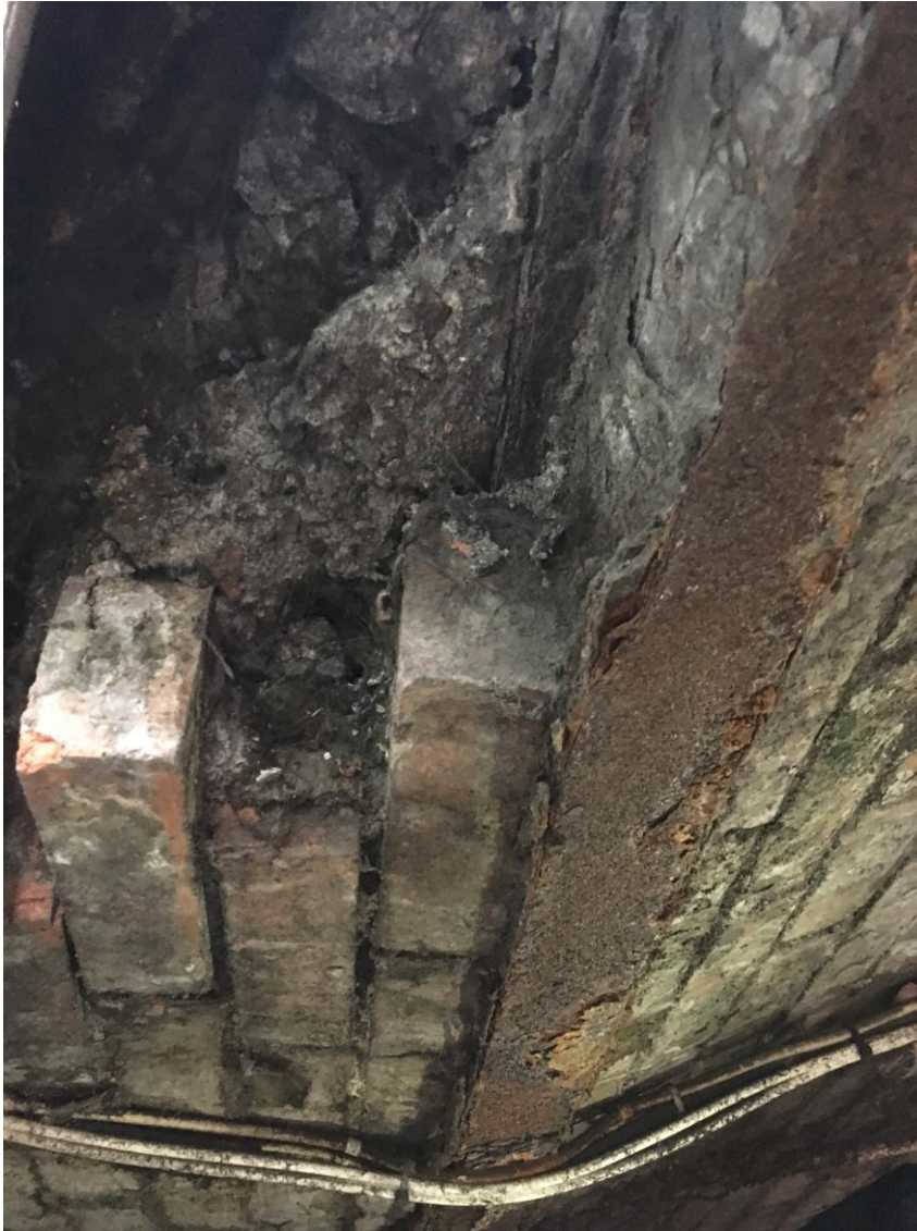
Underside of walkway showing the critically poor condition of the beams
