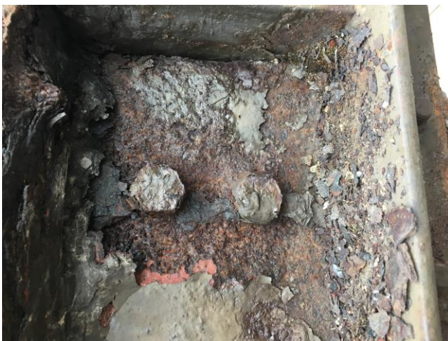
Underside of walkway showing the critically poor condition of the beams
