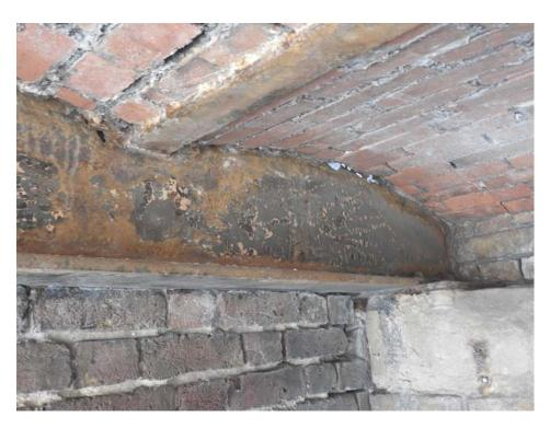
Weaknesses in the existing perimeter secondary beam were observed where the proposed replacement link bridge to the Provender Store is to be supported by the walkway.
