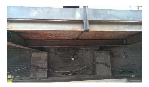
For solutions 3 and 4, the Structural Engineer's proposals include a supporting beam running perpendicular to the reinforcement -beams in the two locations where recently installed gas pipes run alongside the existing primary beam before entering either the Provender Store or the Long Stable.
