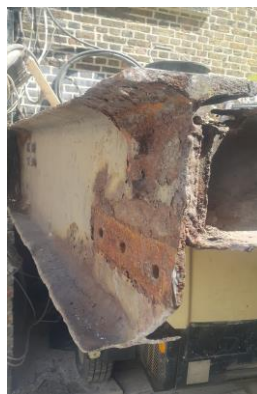
Figure 1: Existing condition of primary beam P1
