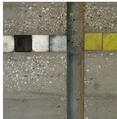
POURED IN SITU CONCRETE - WITH SMALL TILE INSERTS
