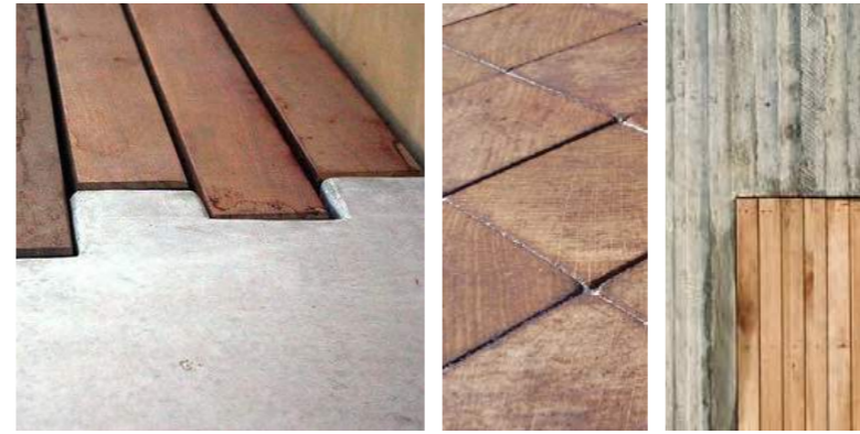
RAISED PLATFORM WITH TIMBER DECKING
