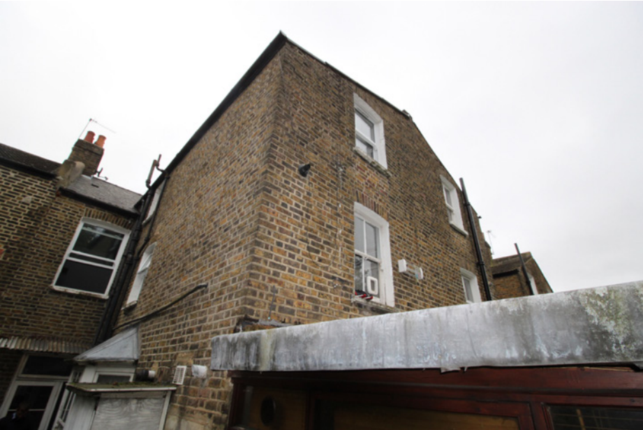
Existing rear outrigger
