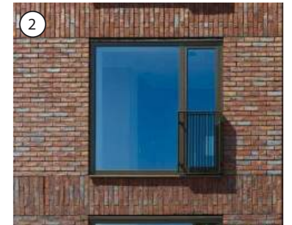
Warm-toned pale red brickwork - expressed floor zones
