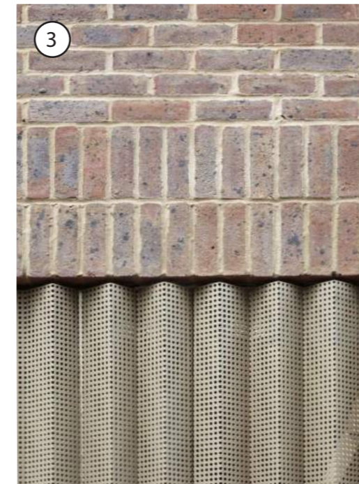
Metal shutter and feature brickwork details
