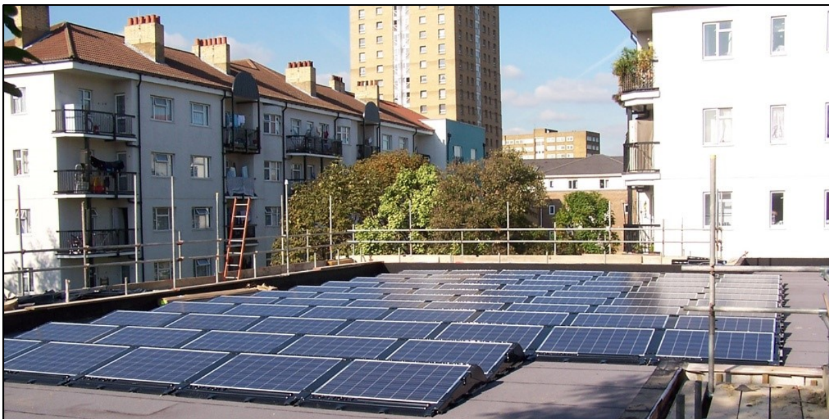
Figure 2 Example of the proposed Low angle PV array.
