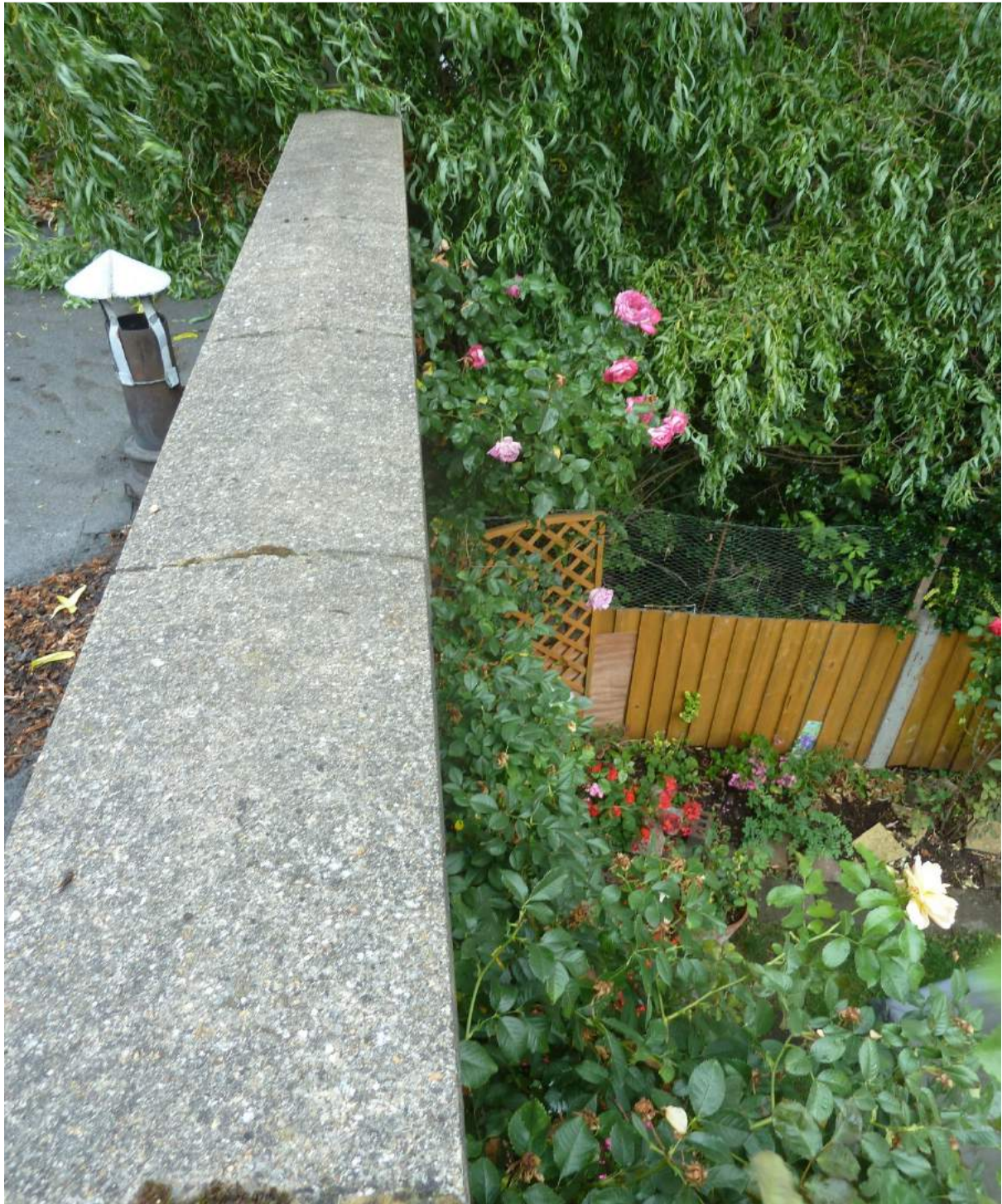
Image 8 View over North Boundary wall into gardens of Collard Place
