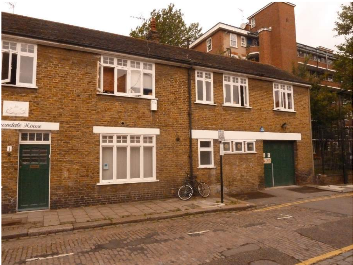
Image 10 East elevation Wall site B
