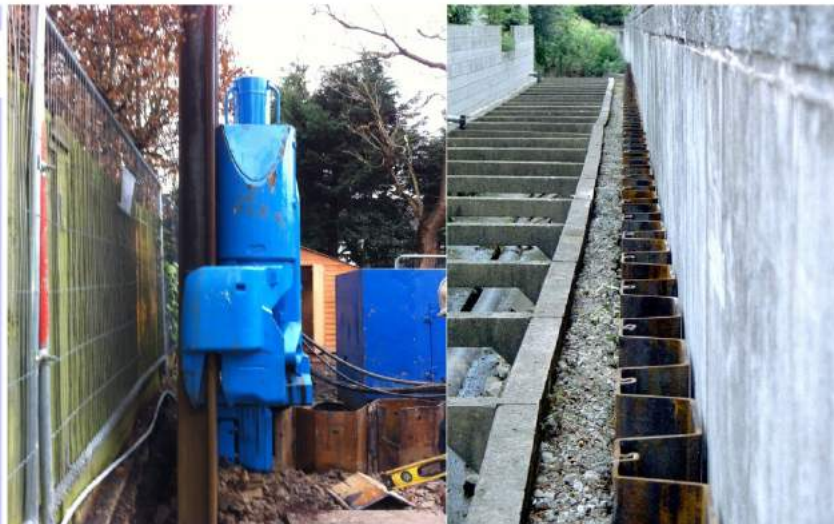
Fig 1 Sheet piling equipment
