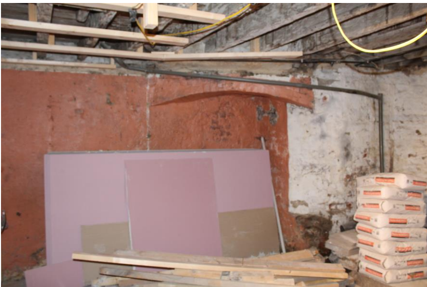
63. Basement support for chimney breast (photo by Laura O'Callaghan Sept 2016)
