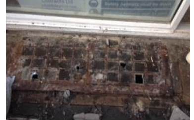
27. Pavement lights prior to removal
