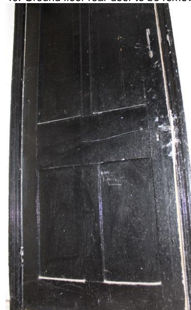
41. Rear ground floor door to be removed
