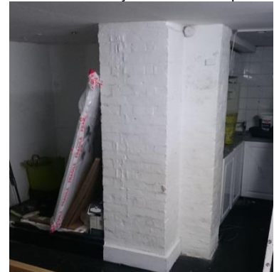
20. Brick pier to be removed
