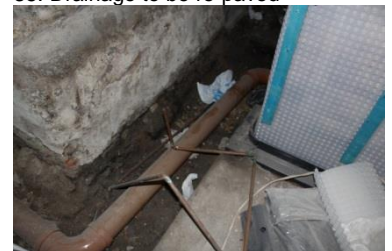
36. Basement tanking in progress
