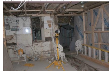
10. Basement looking towards vaults
