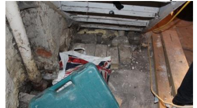
67. Underside of rear staircase
