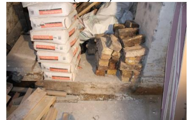
24. Basement floor to be levelled and pier to be removed
