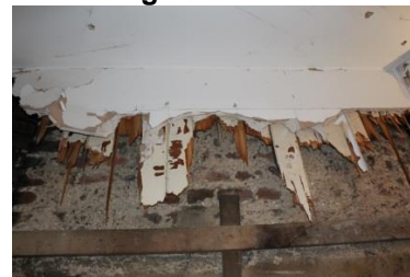
38. Ground floor opening up to inspect rear fireplace structure
