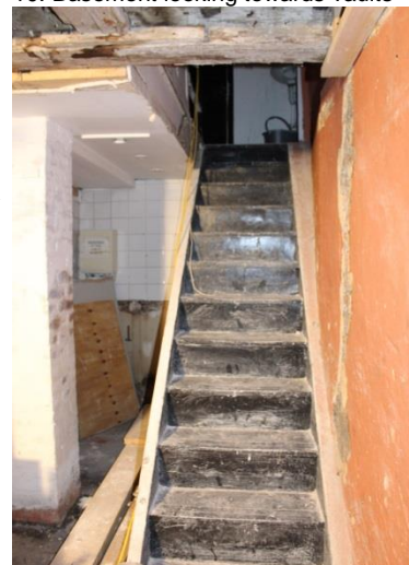
11. Basement rear staircase
