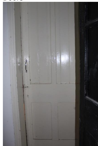
40. Ground floor rear door to be removed
