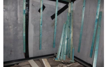
33. Tanking in progress in basement
