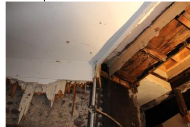
39. Opening up to inspect beam
