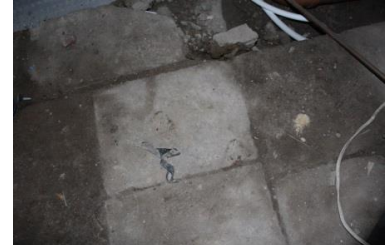
43. Vault Arch 2 paving flagstones
