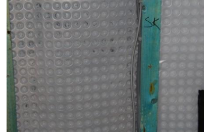
32. Tanking system detail
