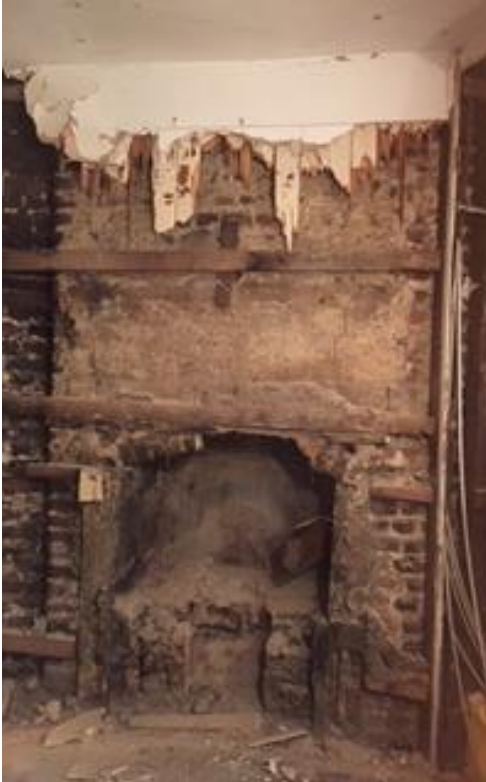
59 - 62. Rear ground floor chimney breast to be repaired (Nov 2016)
