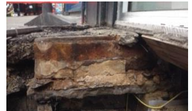
30. After removal of pavement lights
