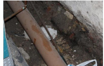
35. Drainage to be re-paved
