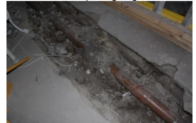
44. Basement drainage excavation
