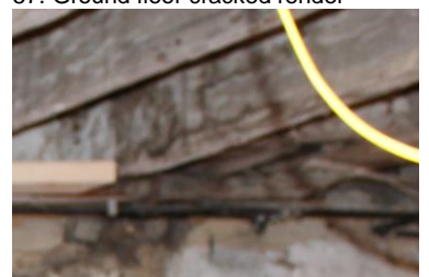
58. Basement ceiling joists
