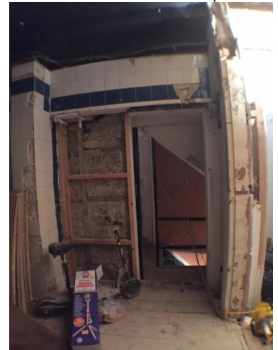
23. Basement pier & partition to be removed And staircase (beyond)
