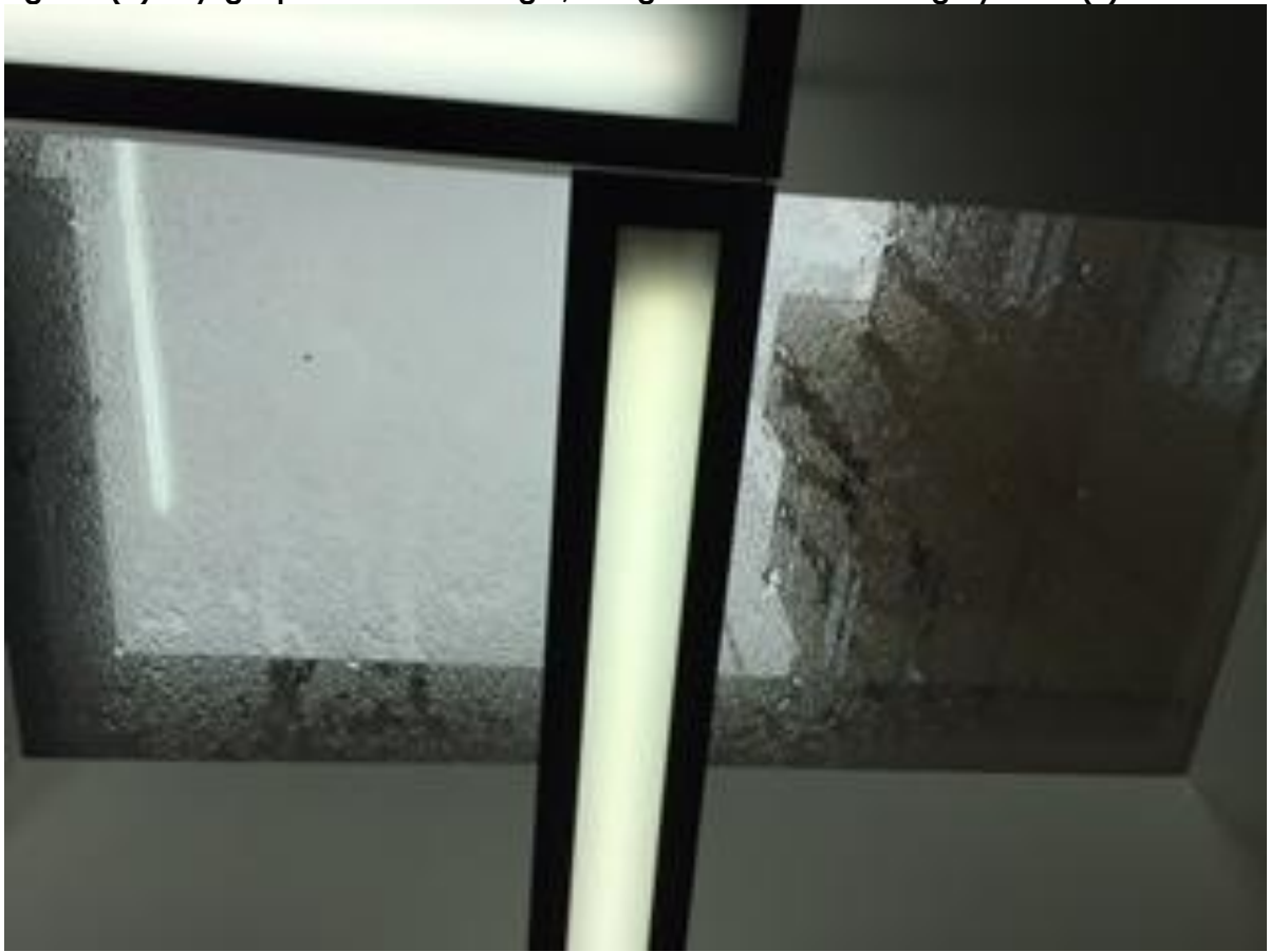
Figure 6(a): skylight provides natural light, sunlight and outlook in surgery room (1)
