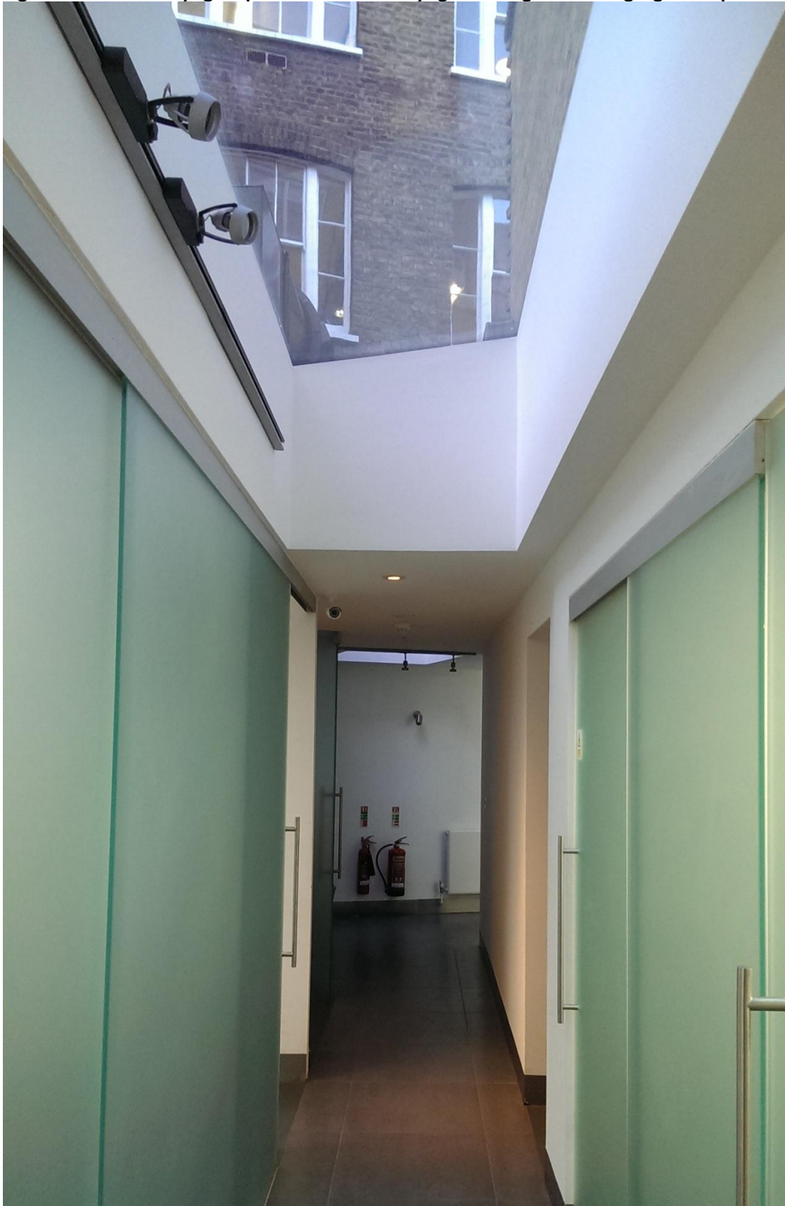
Figure 3: corridor skylights provide natural daylight to surgeries though glazed partitions
