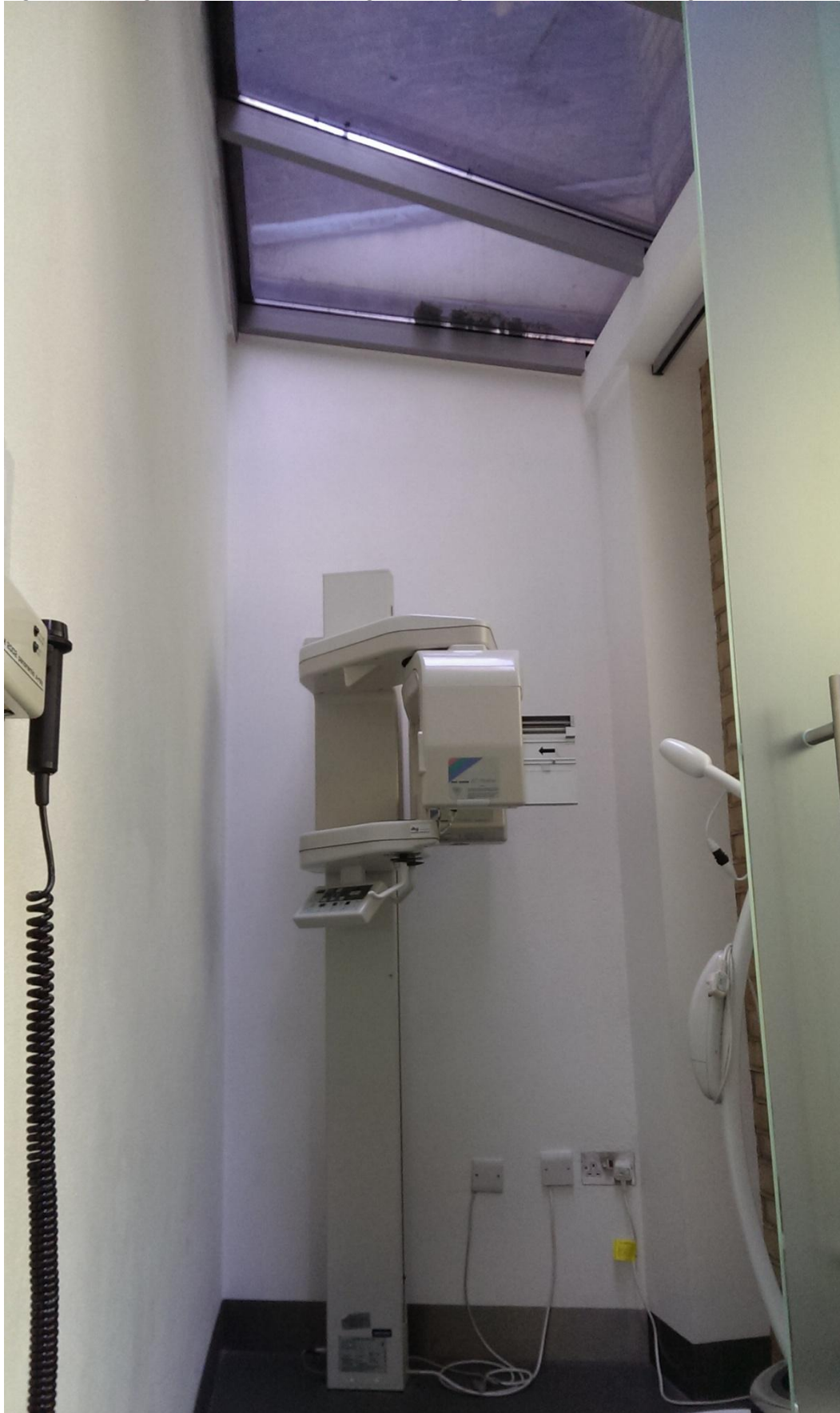
Figure 8: skylight provides natural light, sunlight and outlook for surgery room (3)
