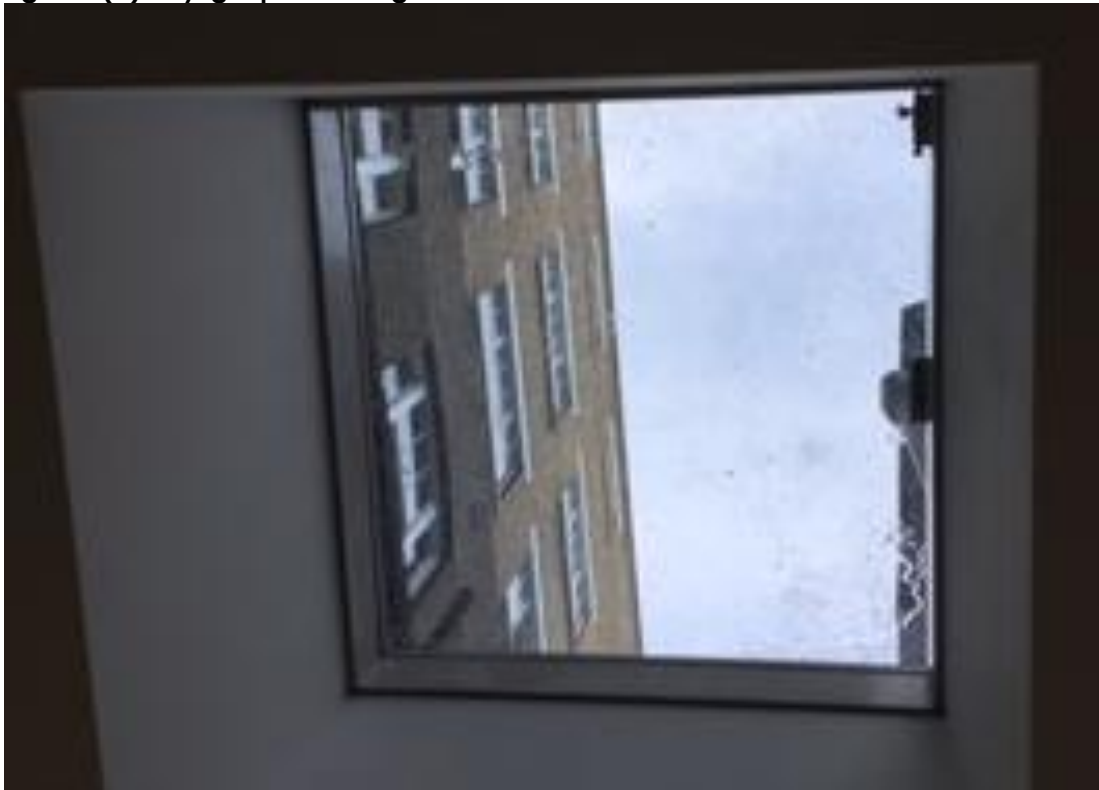
Figure 4(b): skylight provides light to the rear corridor
