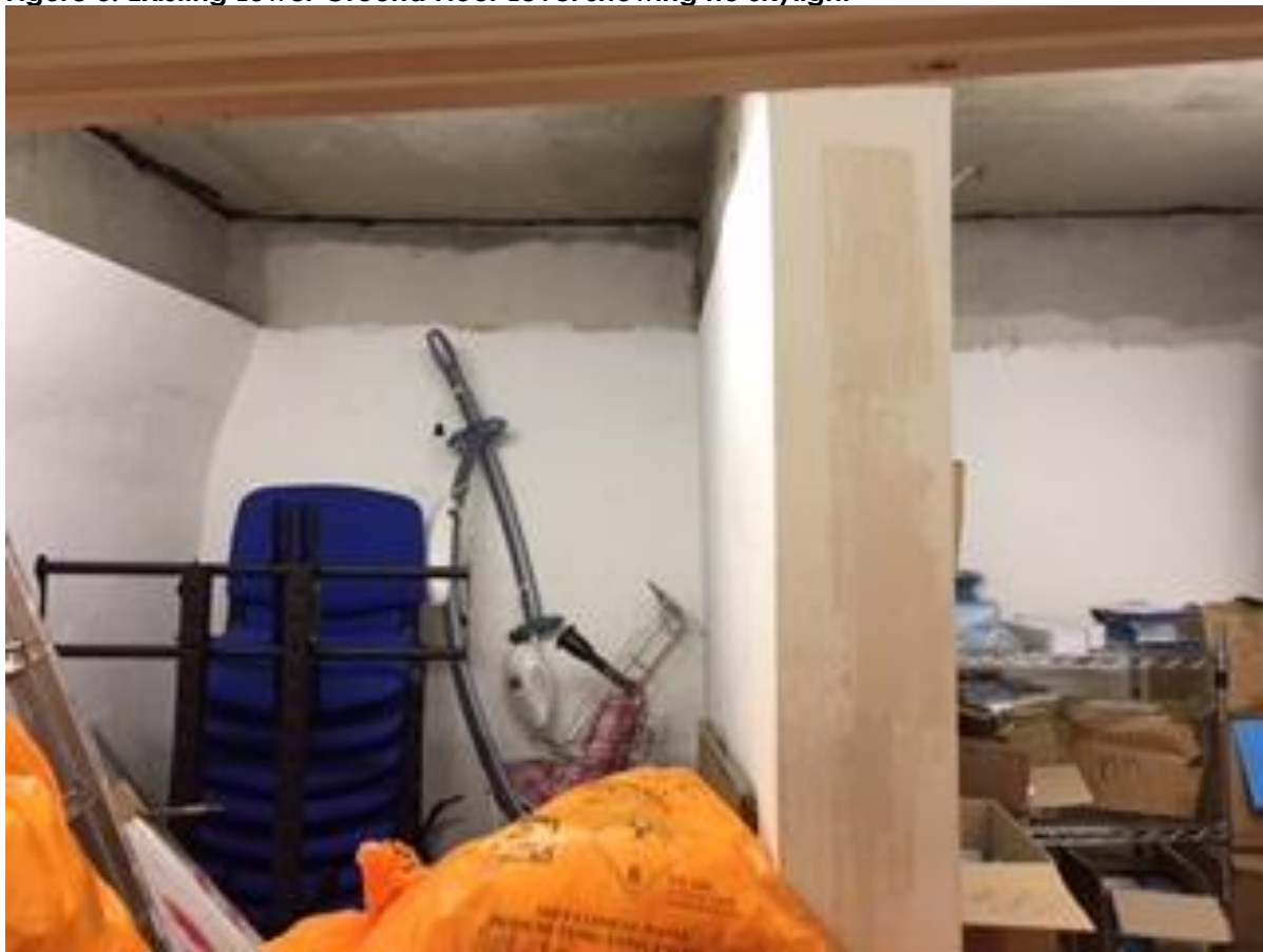
Figure 0: Existing Lower Ground Floor Level showing no skylight
