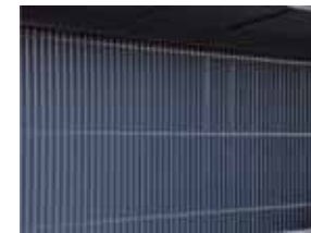
BLACK ARCHITECTURAL METAL LOUVERS RUNNING VERTICALLY
