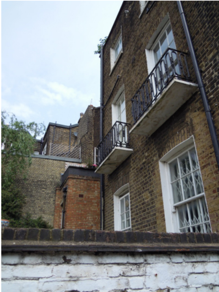
3. rear windows of 1 Highgate Road
