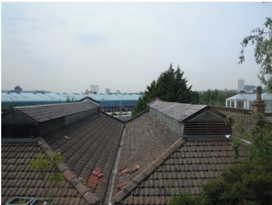
4. View from 1 st floor window of no.1
