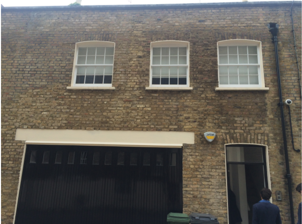
4. Mews rear façade
