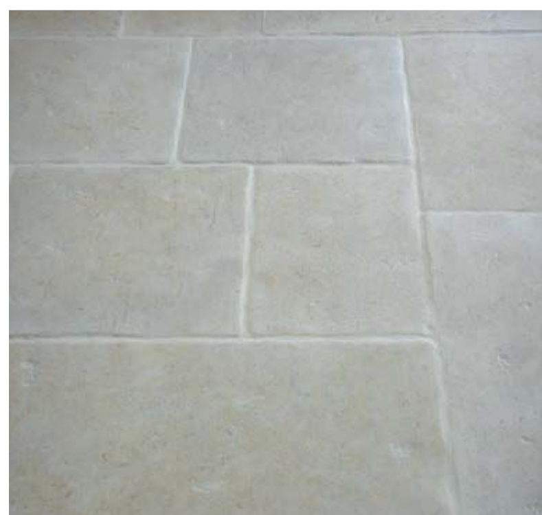
Limestone for the Lower ground Floor
