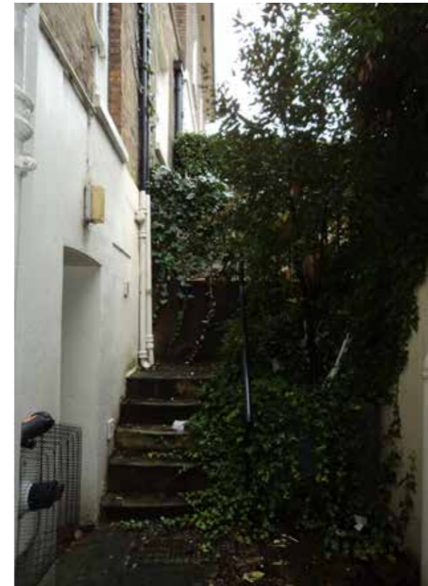
Existing stairs from side footpath to front courtyard
