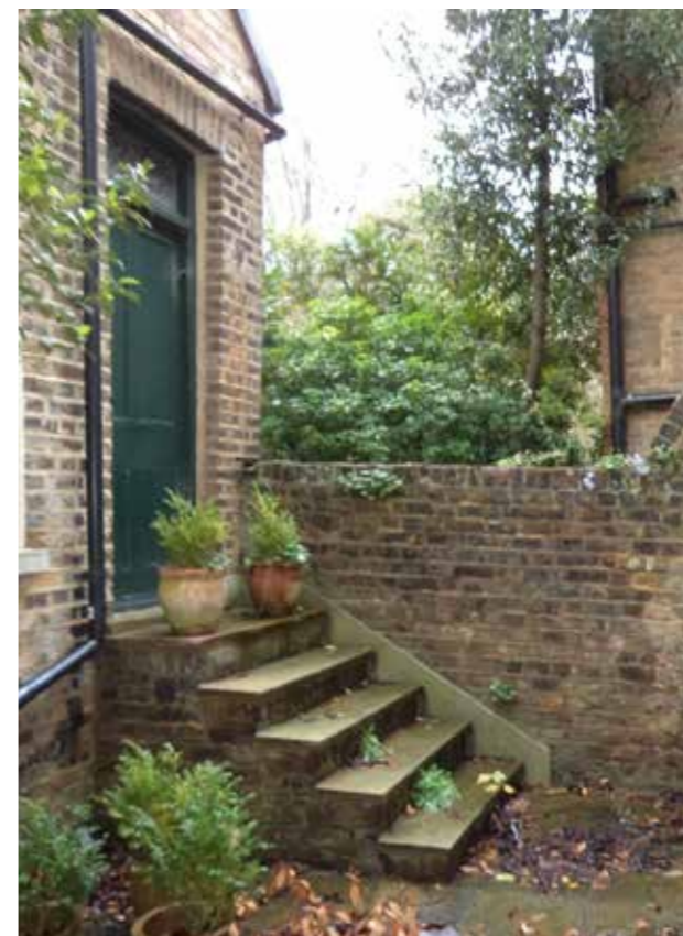
Existing Studio steps
