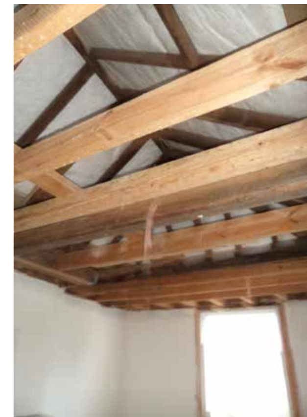
Existing ceiling to stables
