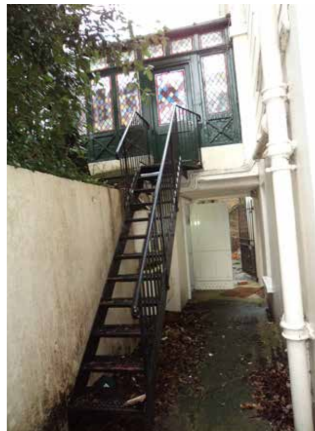
Existing stair in front courtyard
