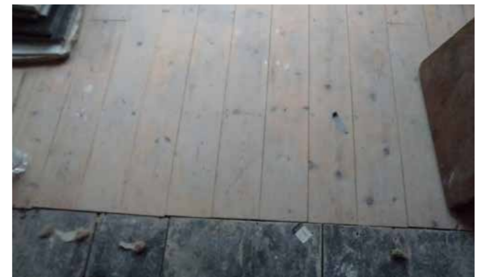
Ground Floor timber floor boards - showing lines of previous extensions
