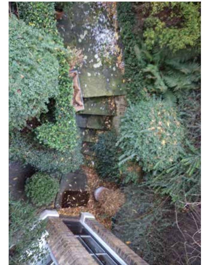
Existing stairs from rear garden to Lower Ground Floor
