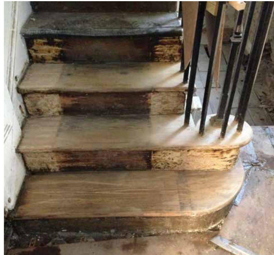
Existing GF bottom steps - Rubber finish removed and surface cleaned
