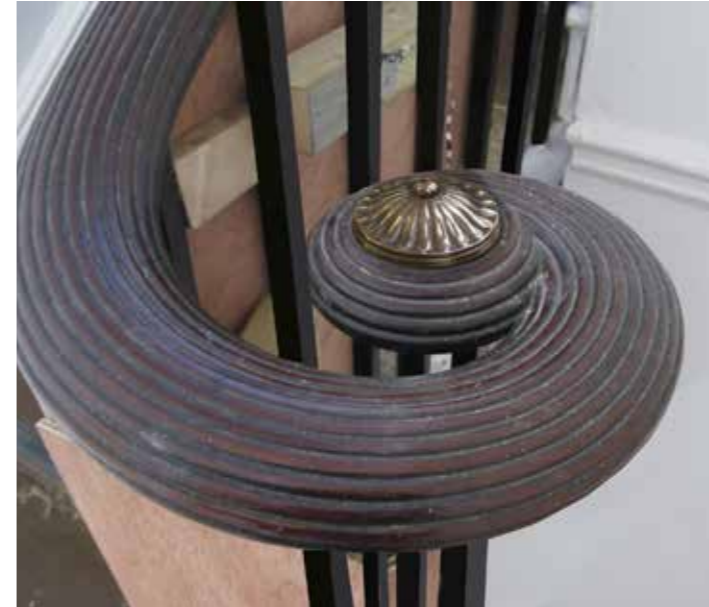
HANDRAIL RAMP FINISH DETAIL IN PATINATED BRASS
