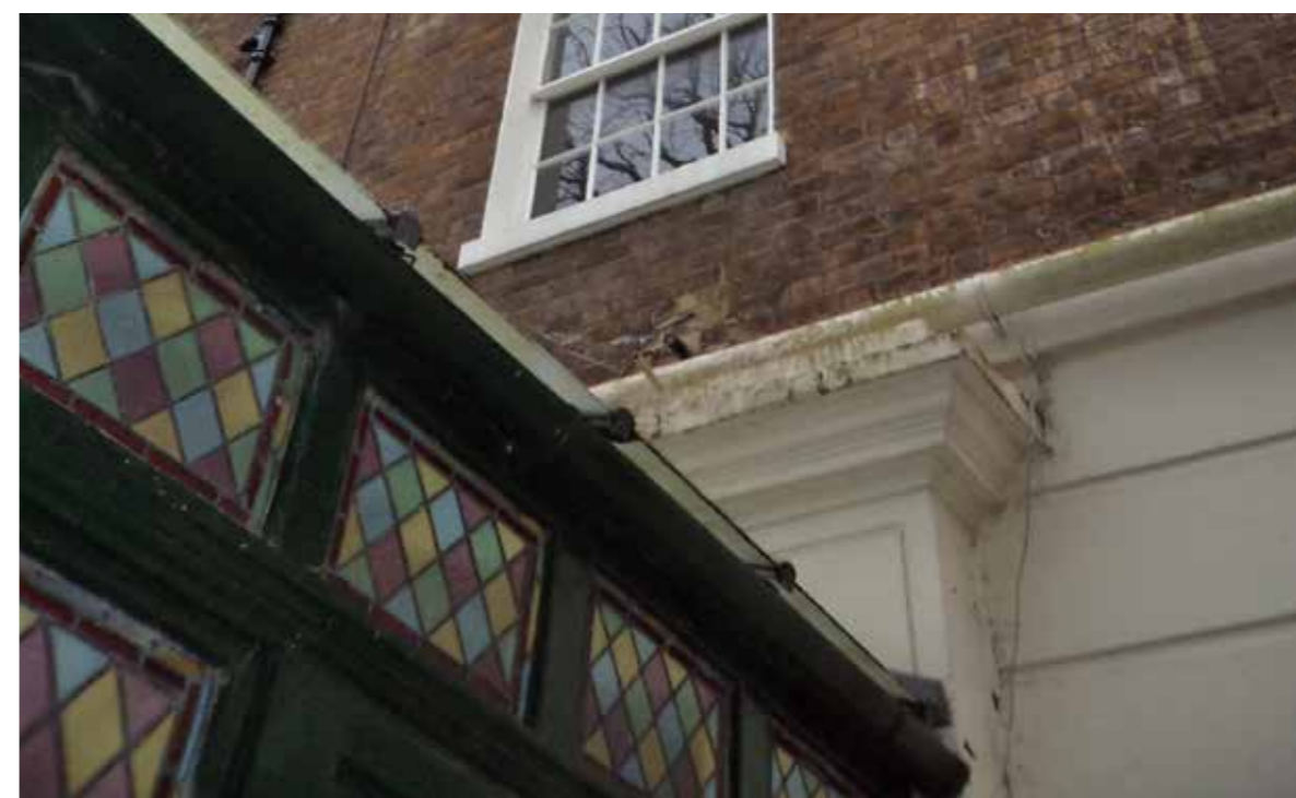
Repairs to brickwork
