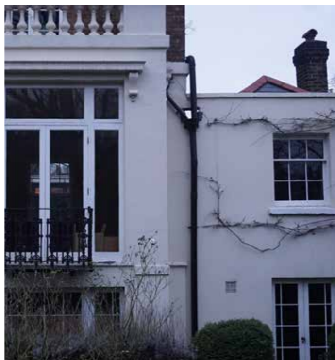
Repairs/rationalising rainwater goods
