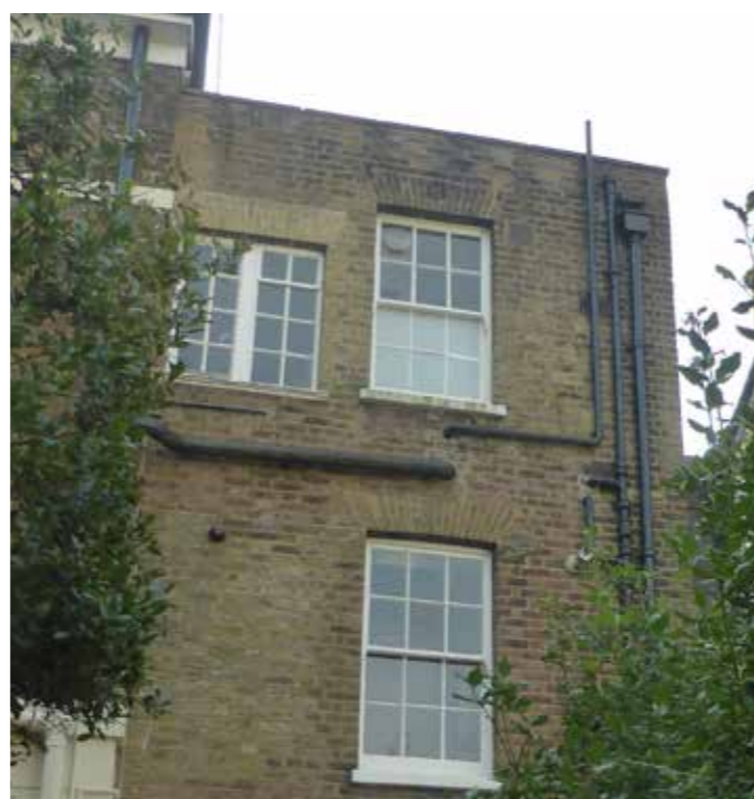
Repairs/rationalising rainwater goods
