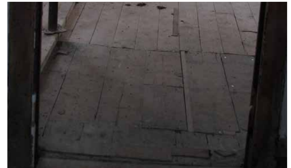
Ground Floor timber floor boards - showing lines of previous partitions
