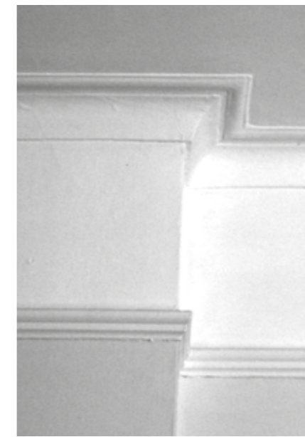
EXISTING CORNICE 10-03 GUEST WC 10-04 SMALL KITCHEN
