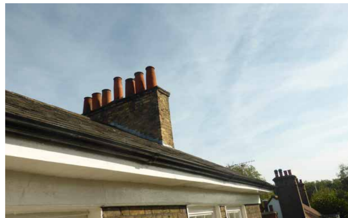
Repairs to gutters
