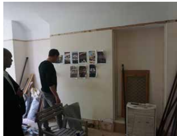
4 storey extension - Chimney to be removed, minimal depth and no longer readable as a chimney breast
