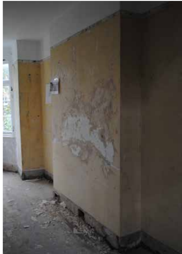
4 storey extension - Chimney to be removed, currently blocked up
