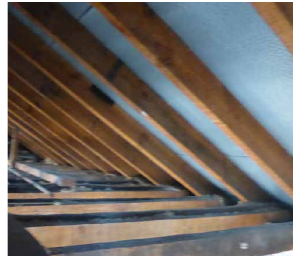
Existing ceiling insulation, joists, rafters and membranes
