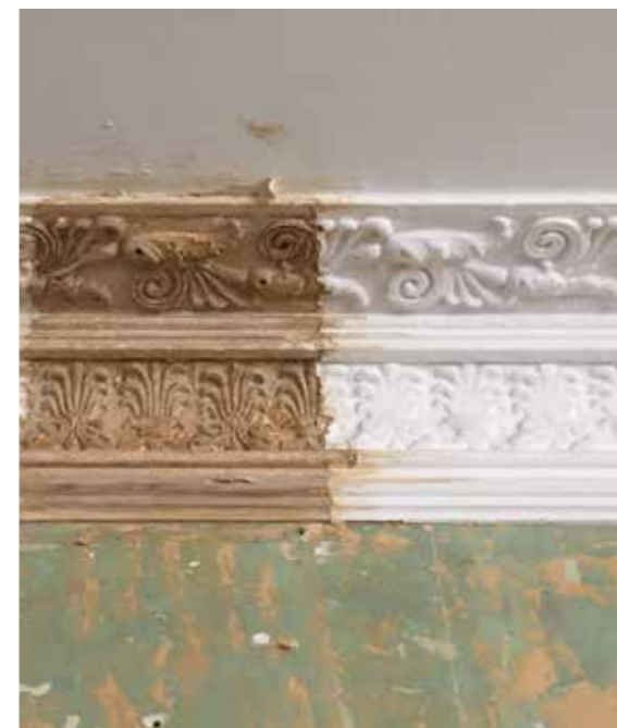
Existing cornices to reception room and lounge to be retained (frieze to lounge to be replaced)- photos show small areas that have been carefully cleaned to reveal the detail
