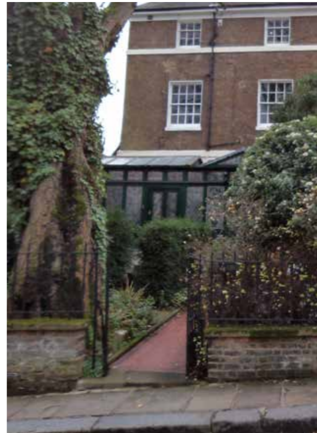
Existing garden wall, railings, gate and tiled pavement
