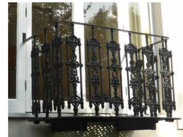
Rear balcony to Ground Floor Lounge; cast iron base and balustrade
