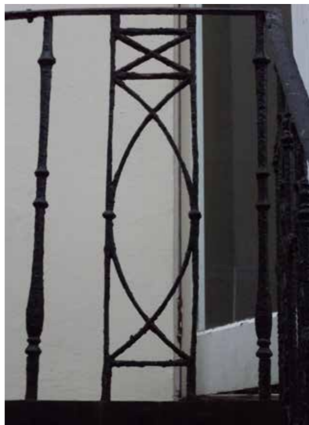
Existing wrought iron detail to balustrade
