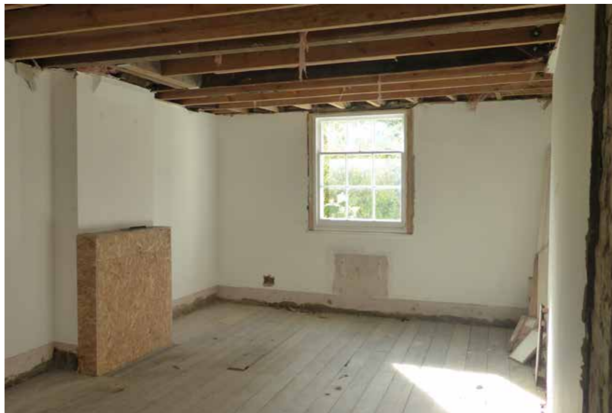
Existing ceiling to stables
