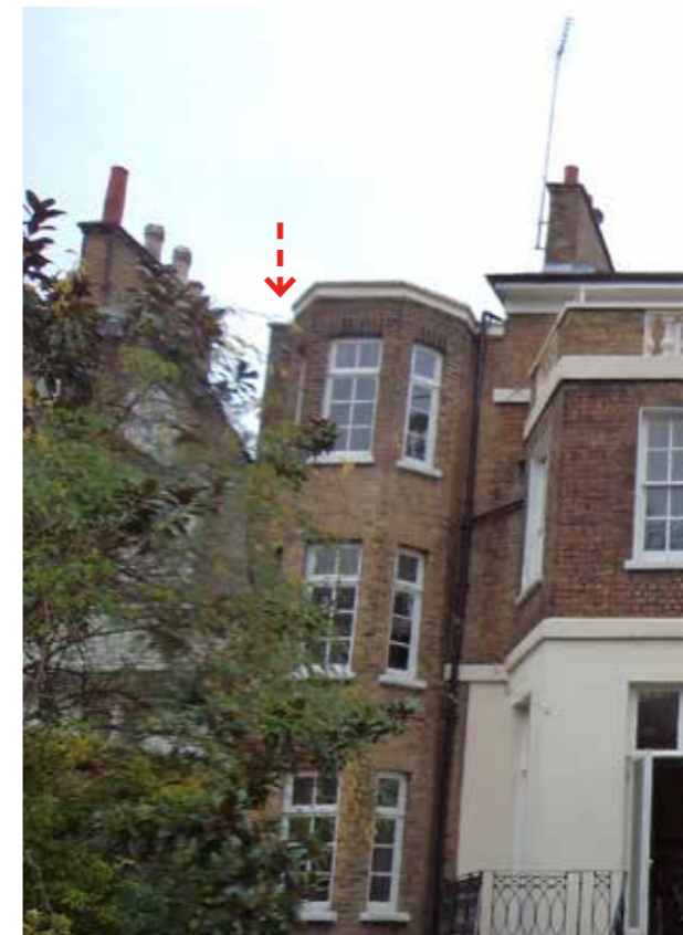
4 storey extension - Chimney not visible from the rear
