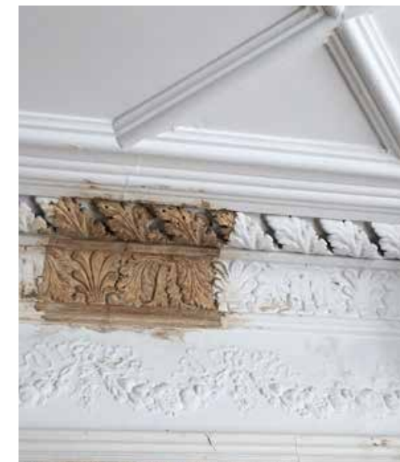
Existing cornices to reception room and lounge to be retained (frieze to lounge to be replaced)- photos show small areas that have been carefully cleaned to reveal the detail
