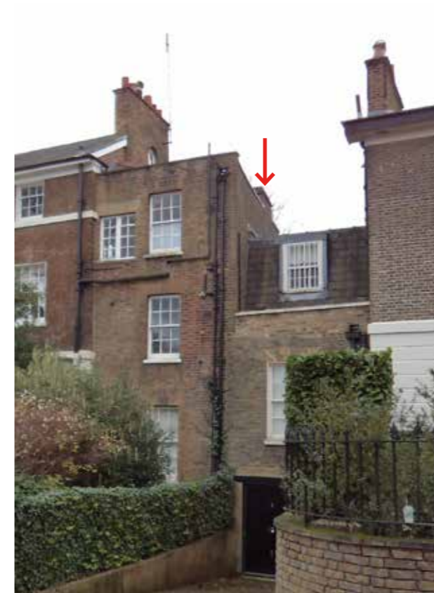
4 storey extension - Chimney to be removed
