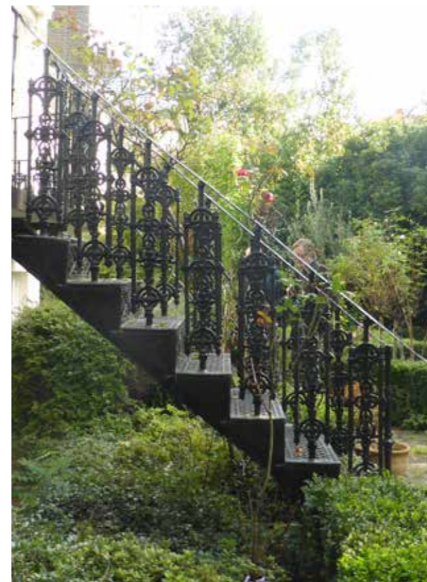
Existing stair with cast iron balustrades
