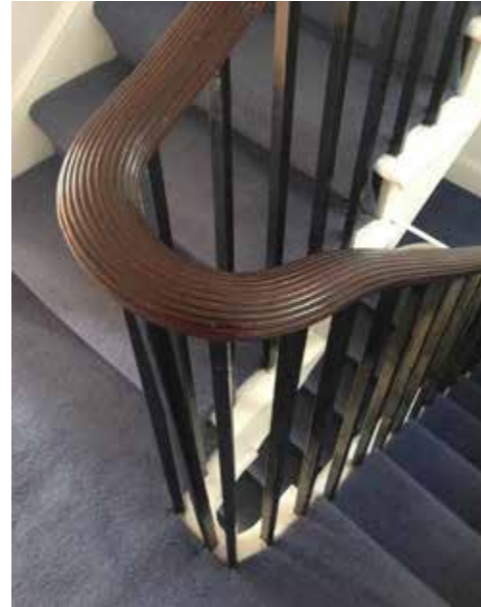
HANDRAIL STAIRCASE AS EXISTING
