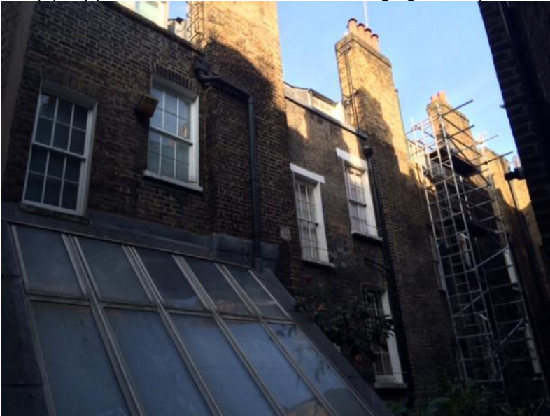
(6) Existing rear lightwell
