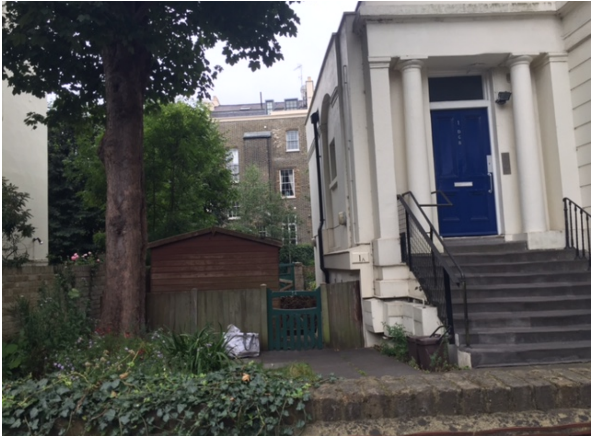
Photo 1 – Close view of front elevation from street
