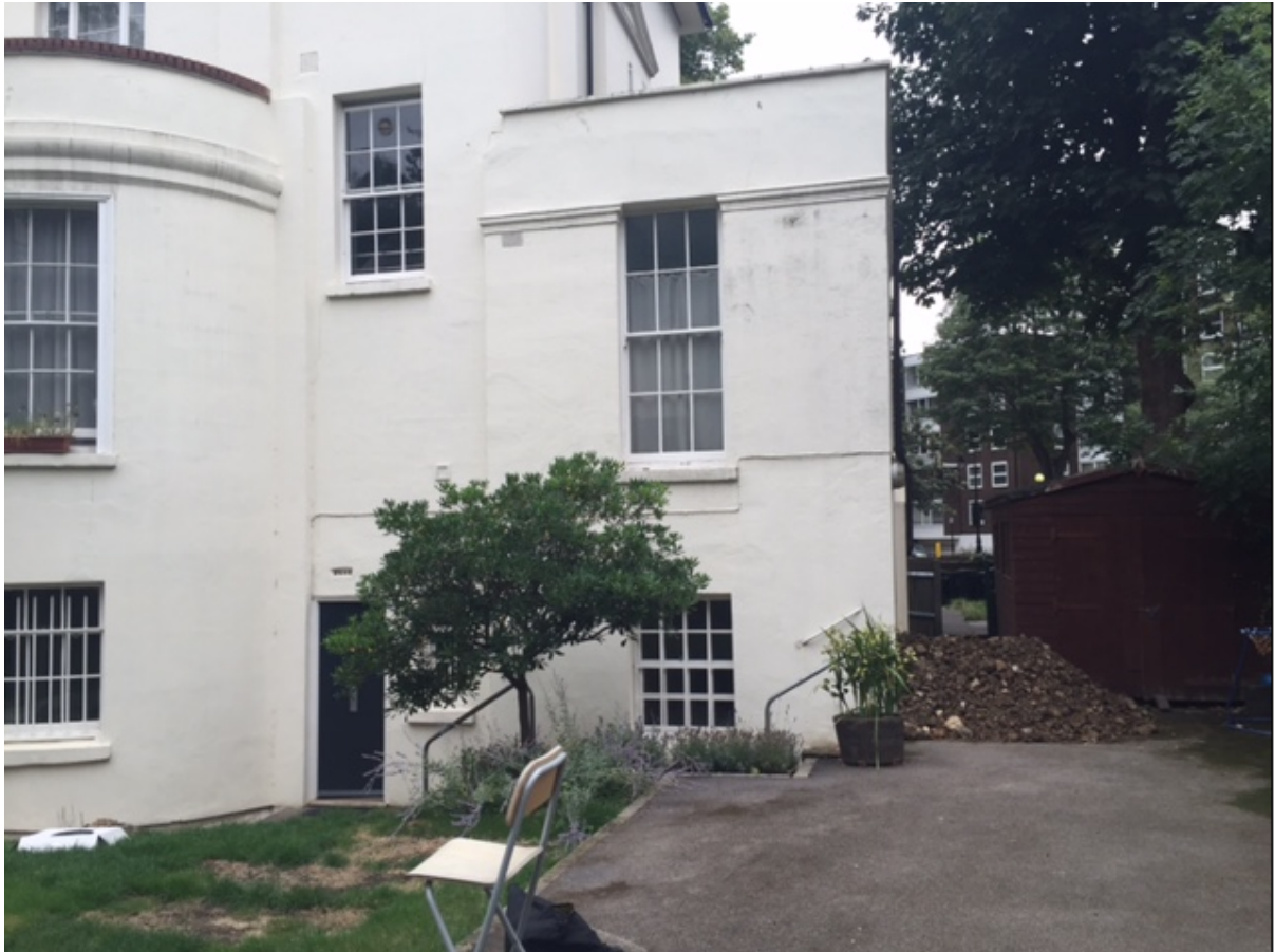
Photo 3 – Close view of rear elevation from garden
