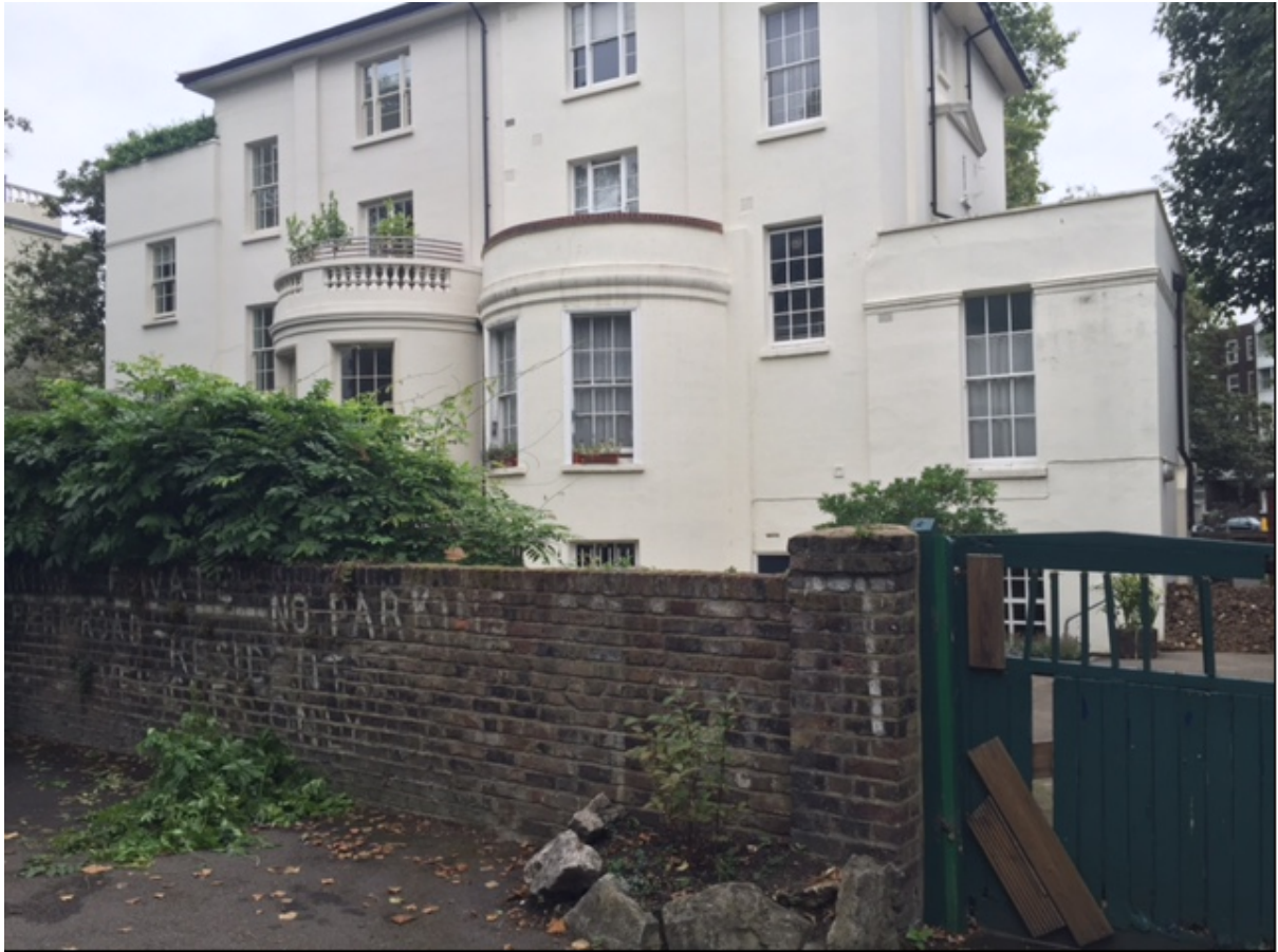
Photo 4 – Longer view of rear elevation from Regal Lane
