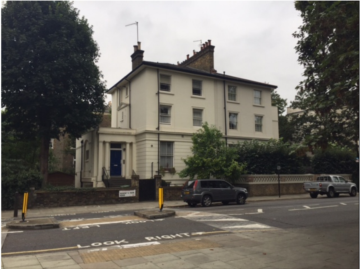
Photo 2 – Longer view of front elevation from Gloucester Avenue/ Regent's Park Rd junction
