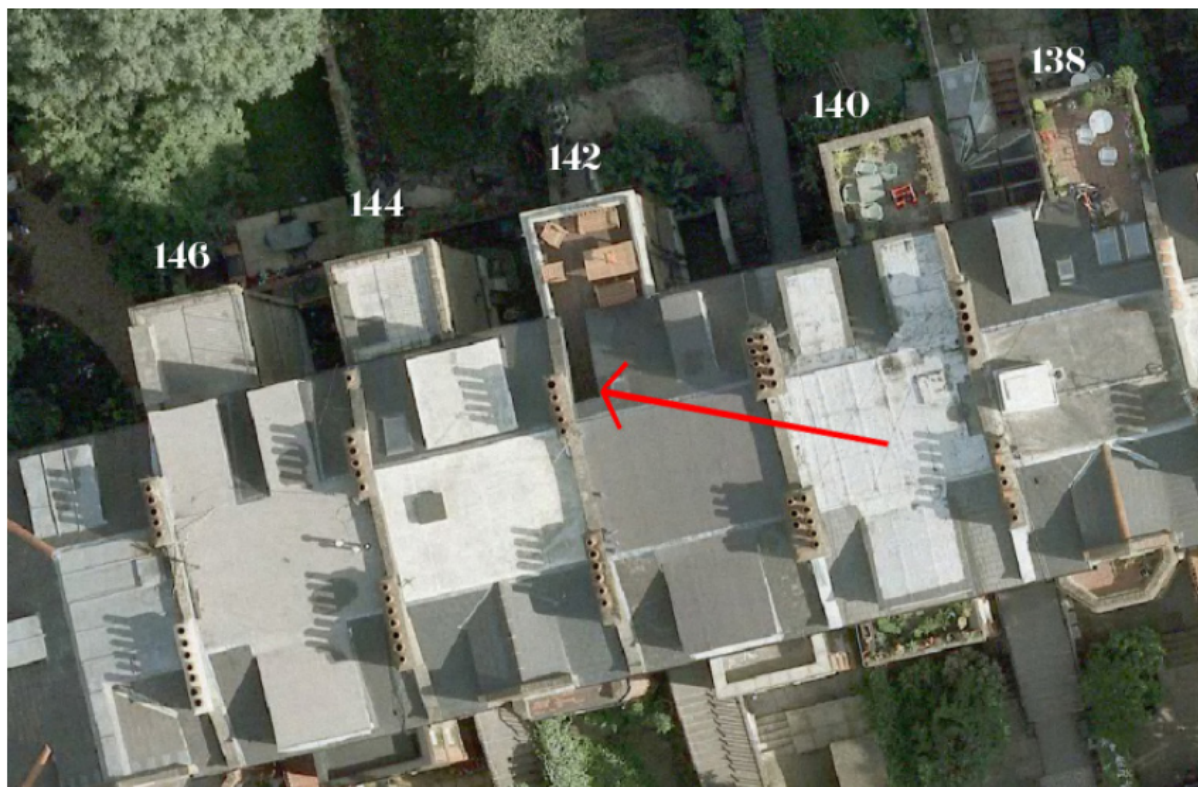
Figure 4 – Aerial view showing similar proposal at adjacent property No. 142 Fellows Road with other roof cut-ins at Nos. 138 and 146 Fellows Road.
