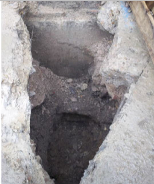
View of FIP02 showing concrete foundation encountered
