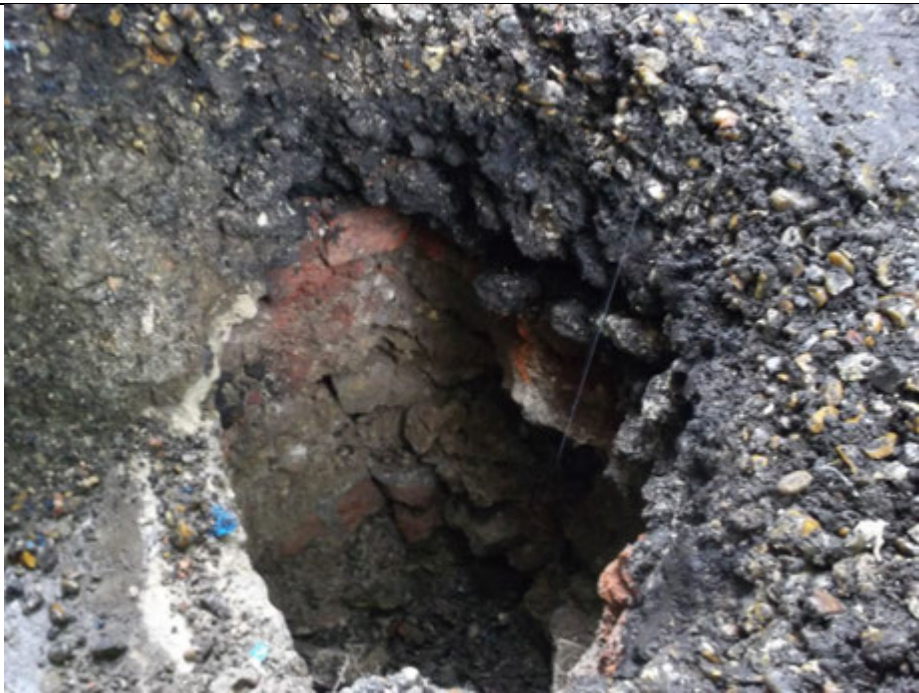
View of Made Ground and concrete footing in FIP01
