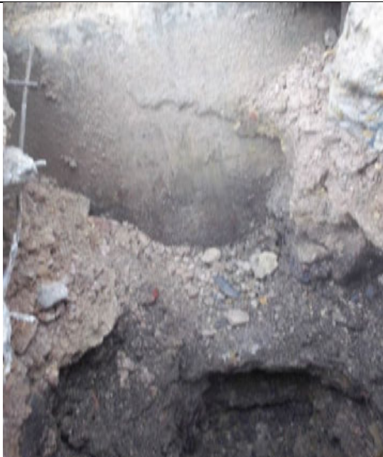
View of Made Ground and concrete footing in FIP01
