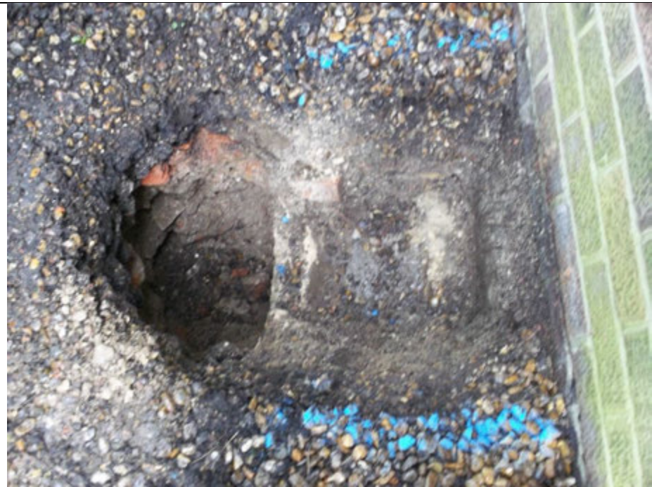
View of concrete foundation encountered in FIP01
