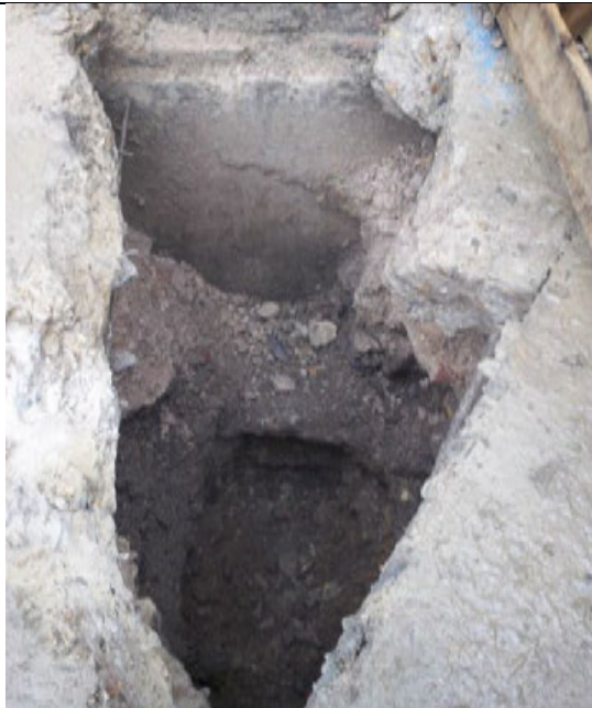
View of FIP02 showing concrete foundation encountered
