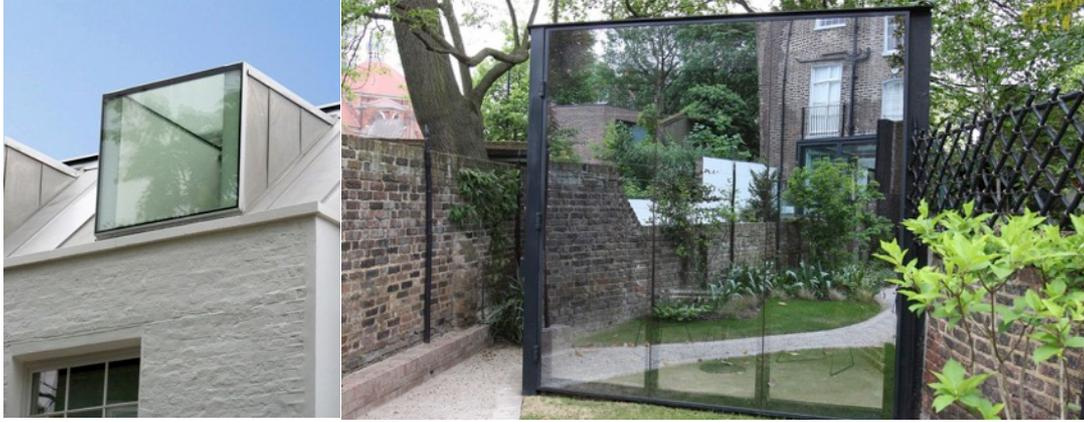
*Fig 3: Examples of glazed lead clad dormer and extension with reflective glazing*
