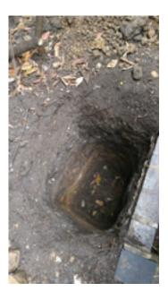
4.1.3 As is evident from the site photographs very limited root activity has been encountered during the hand dug excavations for this trial pit. Even the face of within the trial pit closest to the Hawthorn tree, T3, shows minimal fibrous root growth with no larger anchorage tree roots.
