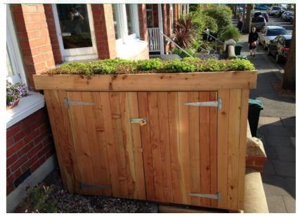
The proposed shed will have the same 'green' roofing and cladding, but will be sized as per the submitted plans. The proposed shed will also feature doors that will slide, one in front of another, rather than (as illustrated above) doors that open outwards.
