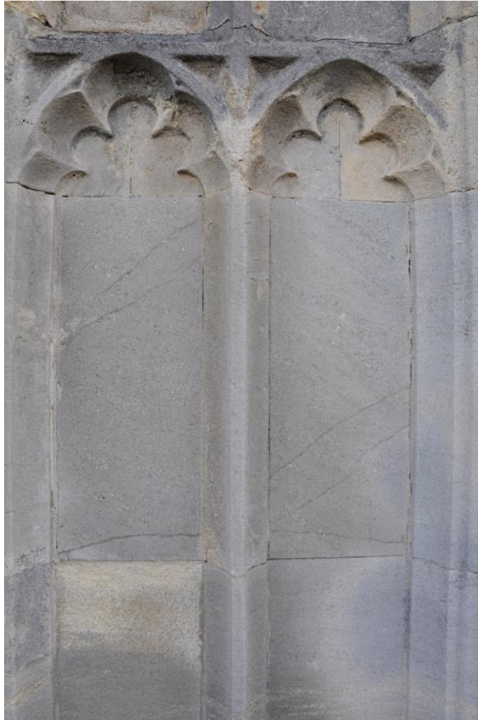
Photo 07 – straight bonded stonework in tracery
