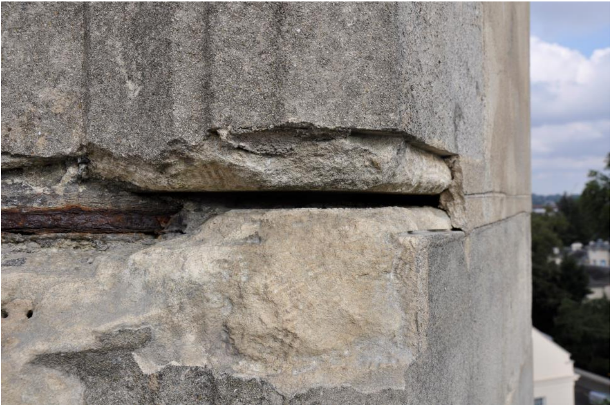
Photo 04 – north tower, parting in bed joint, note later repair to side face masking extent of parting.
