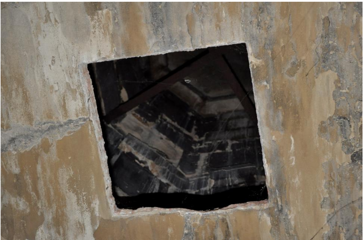
Photo 02 – south tower, looking up inside trceries (note assumed wrought iron brace)
