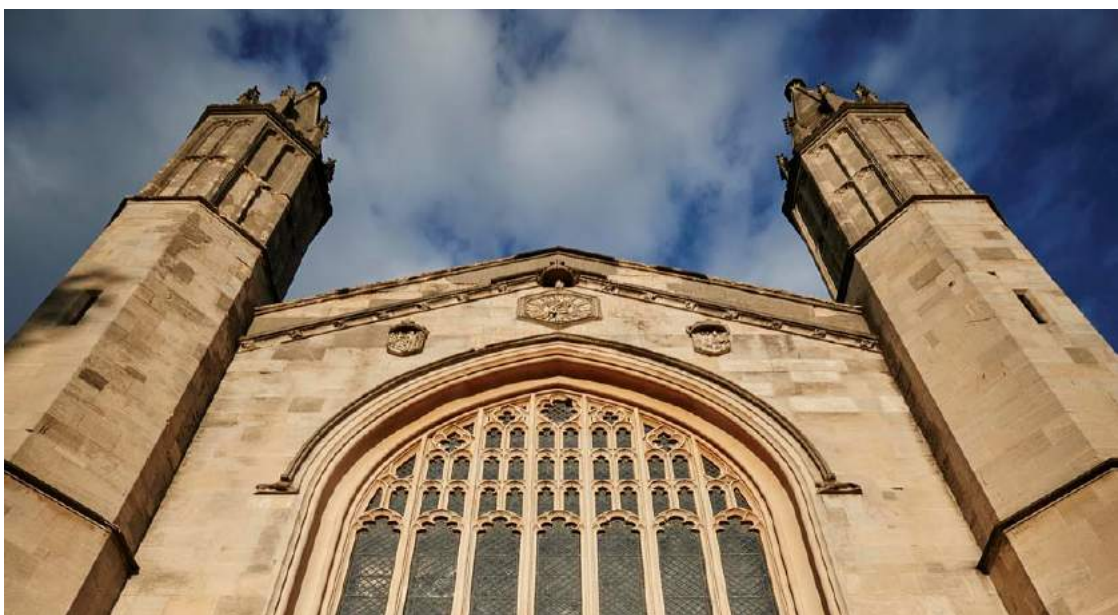
Fig 12. A detail view of the church's west elevation (St Katharine's)
