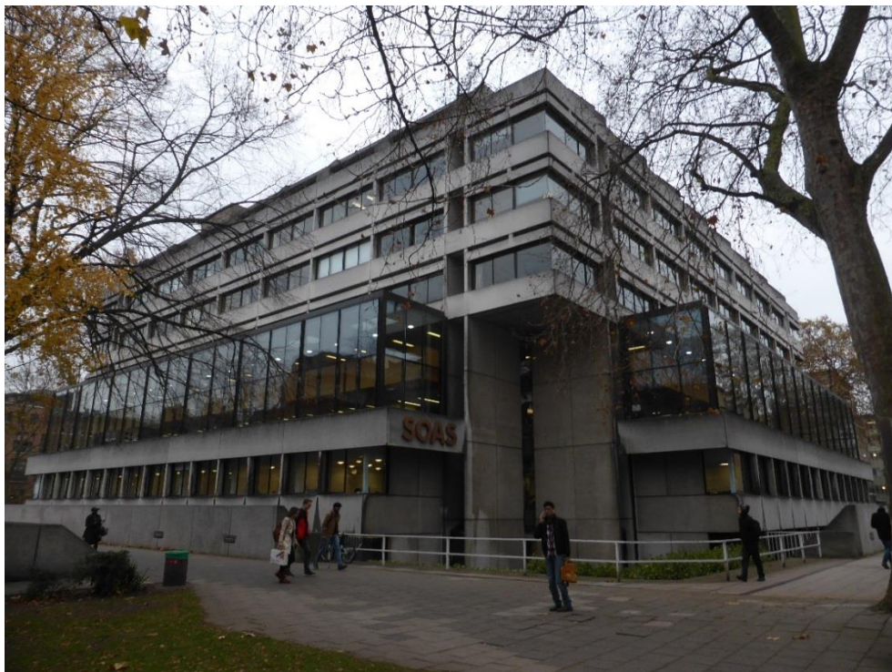
Exterior view of Philips Building
