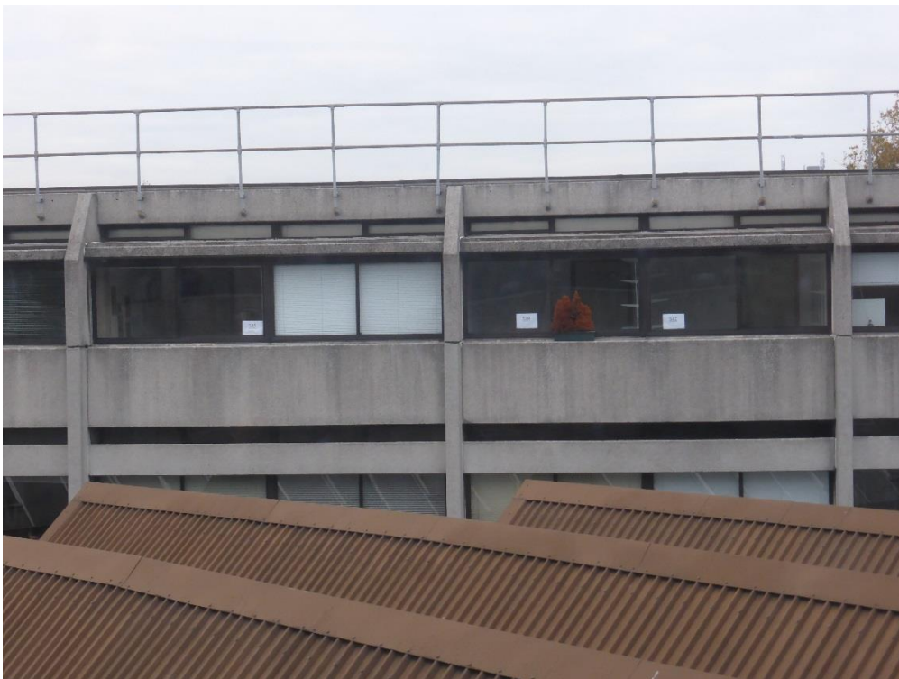
Rooms 535, 539 and 541 (identified with signage), as seen from across the north lit roof
