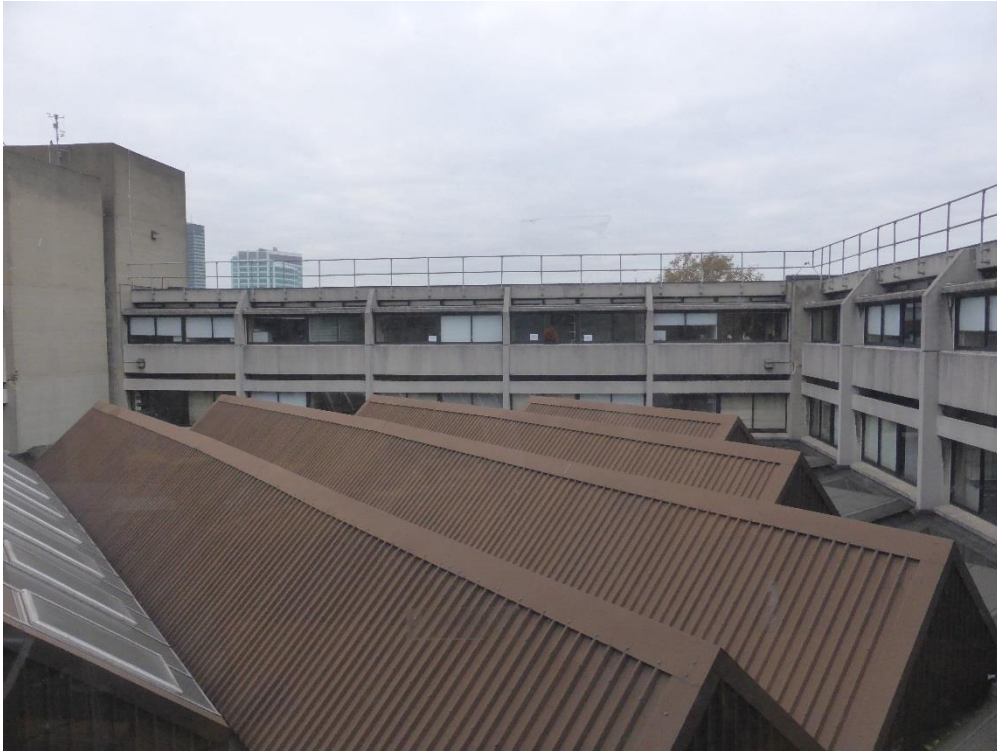
Rooms 535, 539 and 541 viewed from across the north lit roof
