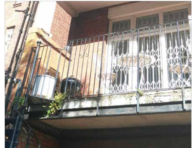
Existing rear terrace balustrade
