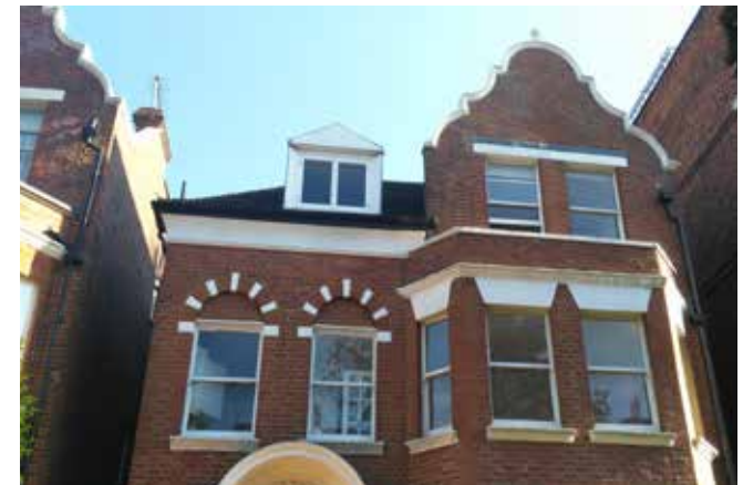
Existing windows and brickwork
