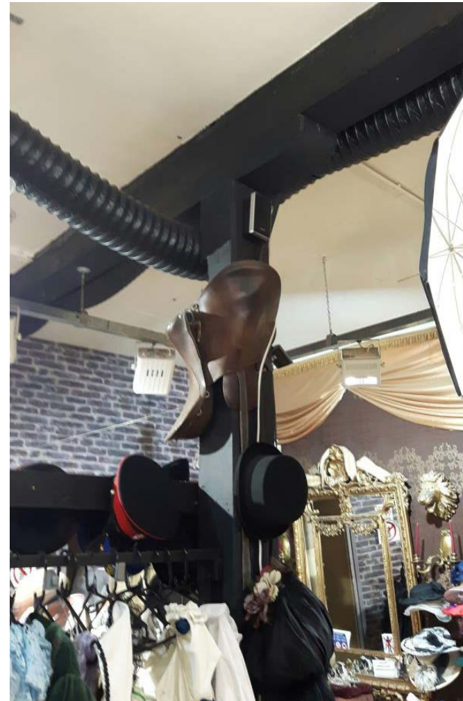
Figure 6: Tack Room: ground floor: north bay. The partitions and wall linings are modern and to be removed. The timber first floor structure and column are original.
