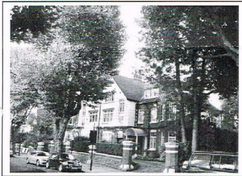
Image of front of property showing T1 on left and T2 on the right.
