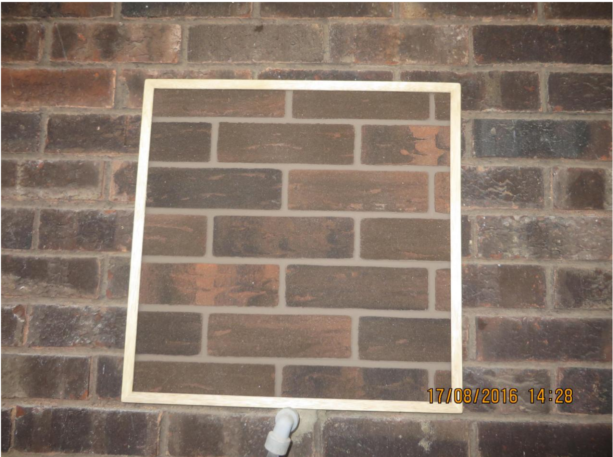
Sample Panel of Sto brick slips in front of existing
