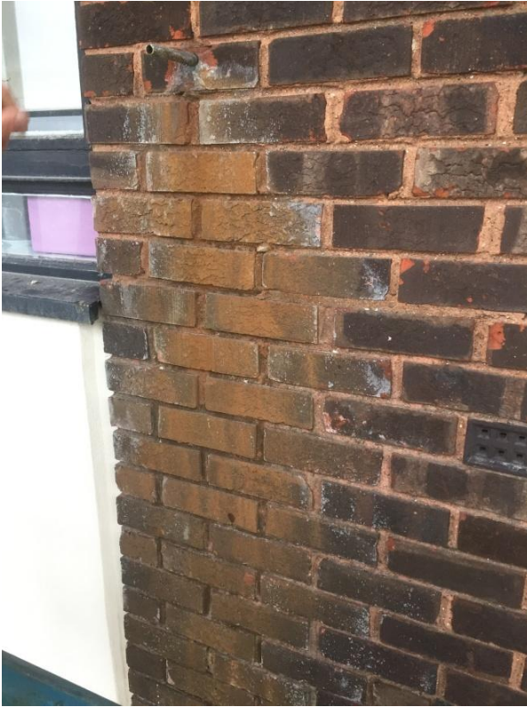
Existing brickwork stained from WC overflow pipes
