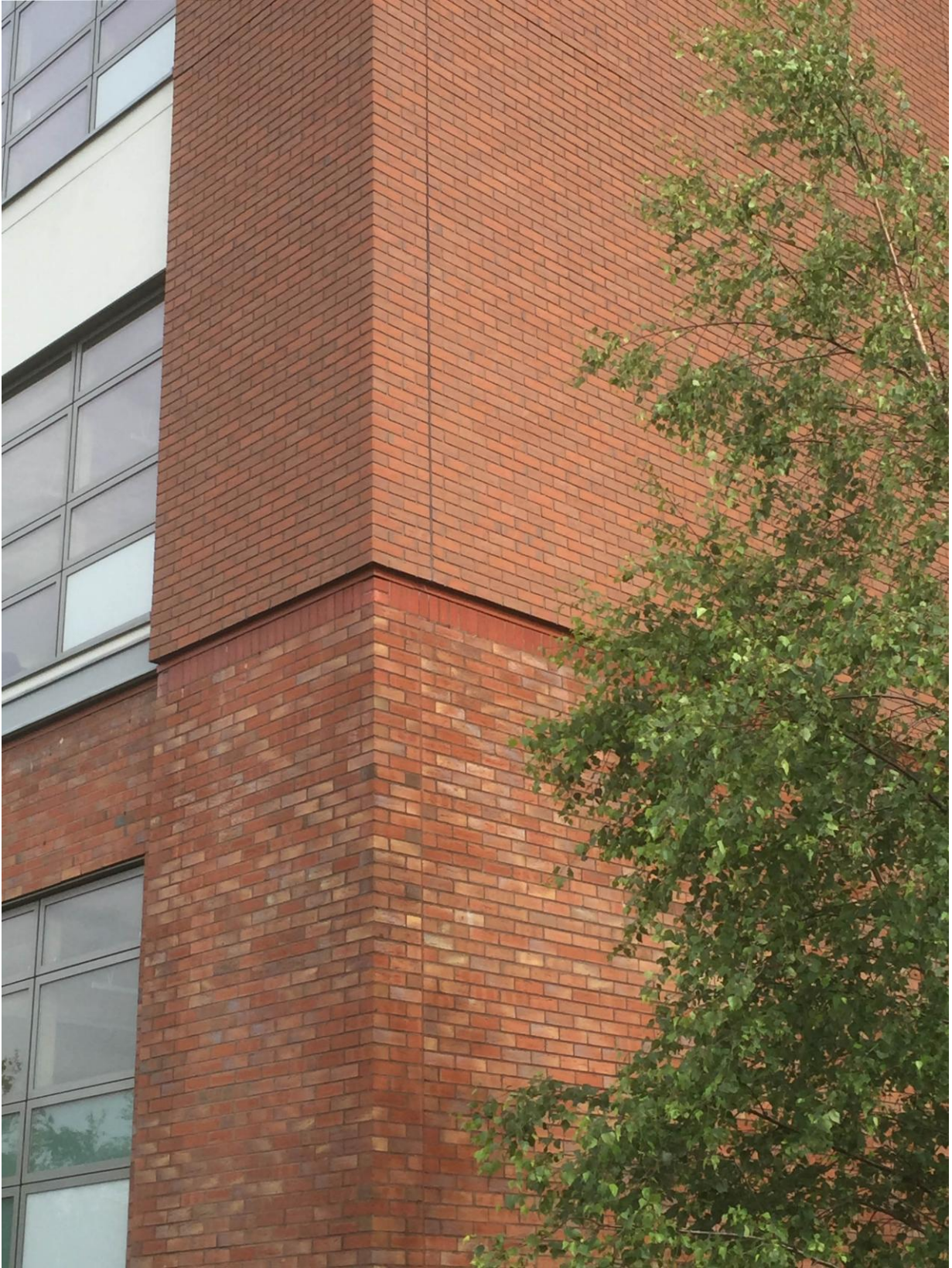
Sto brick slip cladding as replacement for failed clay brick slip cladding
