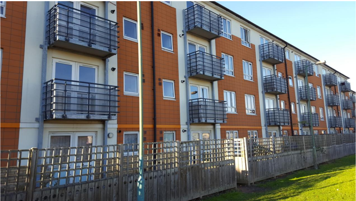
Sto brick slip cladding as of November 2016
