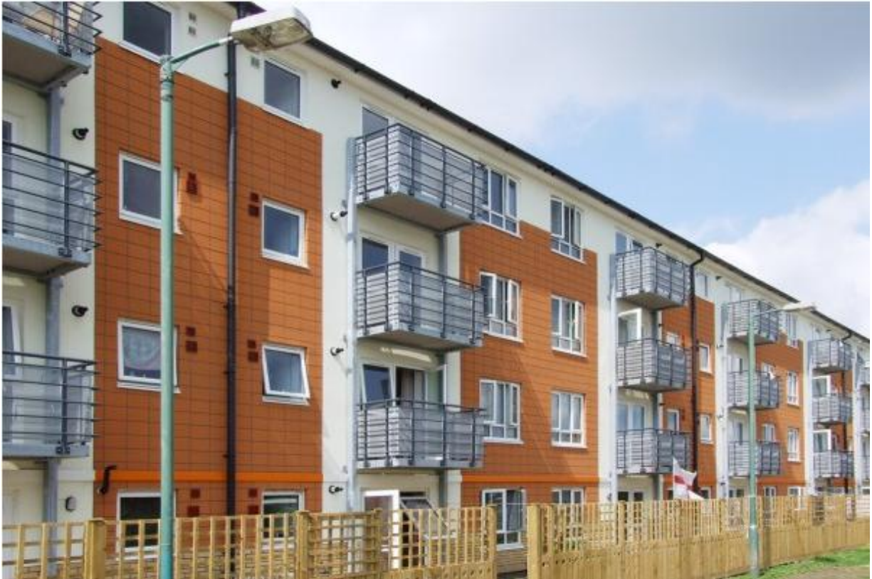
Sto brick slip cladding when completed in August 2009
