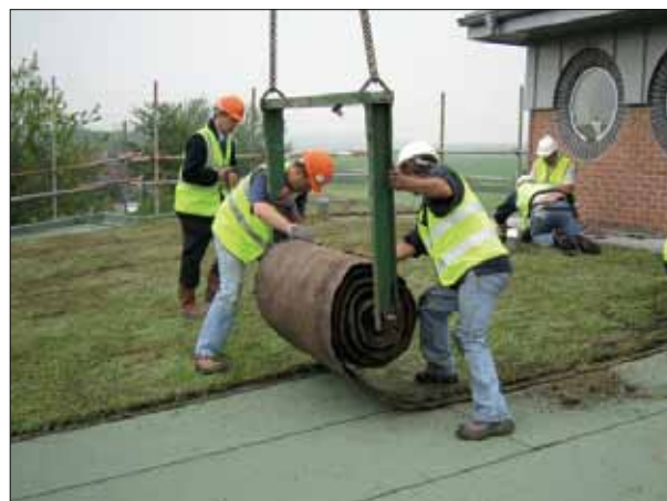
▲ Long length rolls being craned into position and installed.
