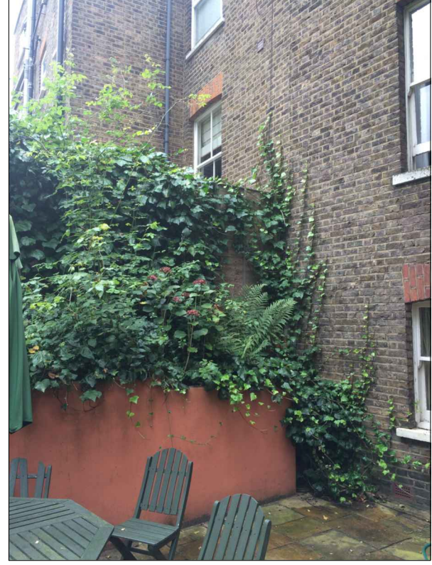
EXISTING MASONRY AND TIMBER GARDEN WALL ON A BOUNDARY WITH NO 23 KINGDON ROAD, APPROX HEIGHT 3.6M
