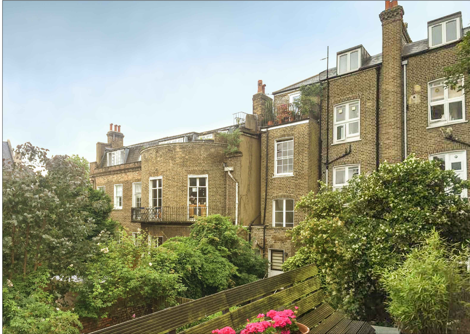
View from the rear as existing
