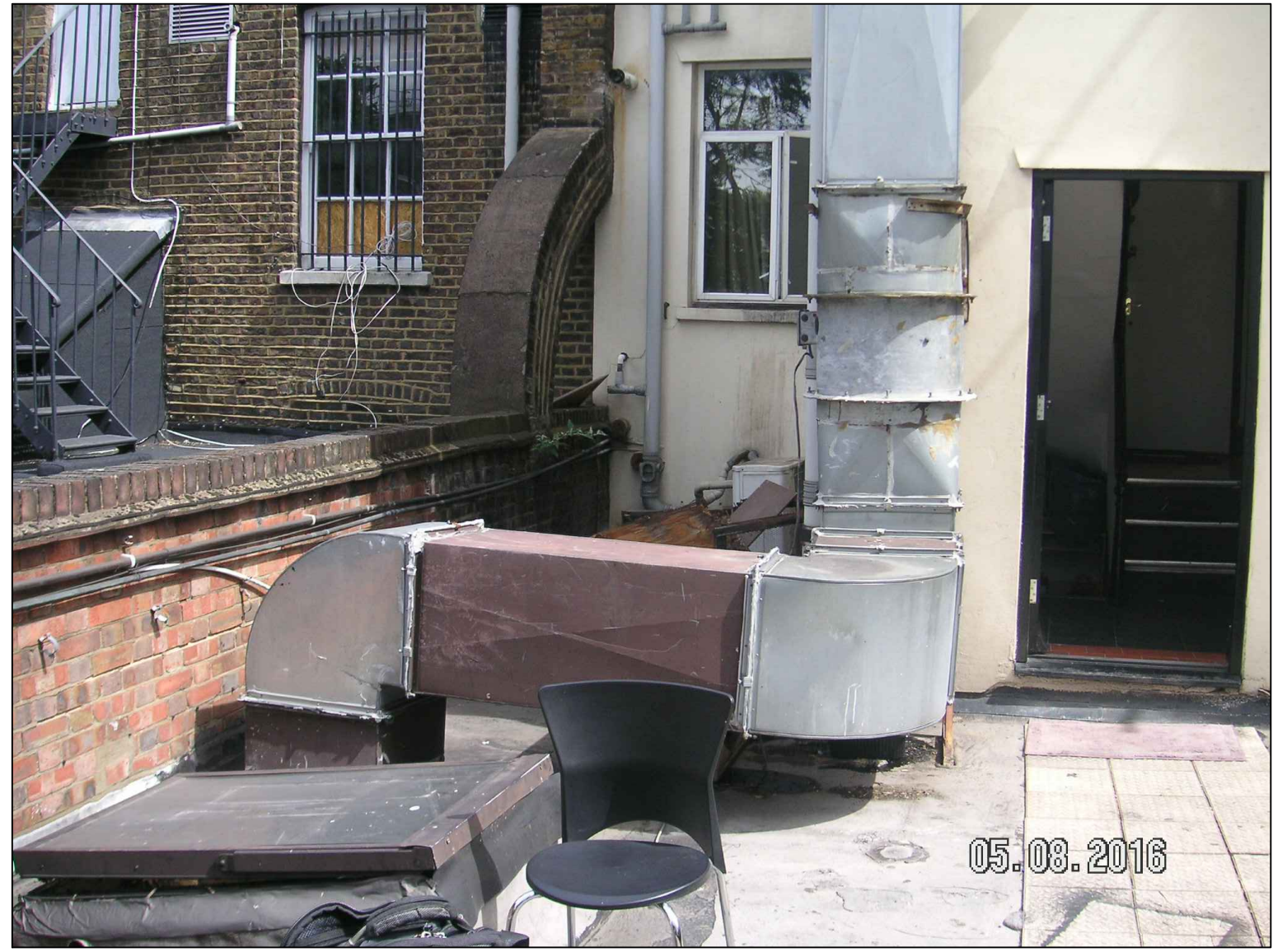
existing rear elevation photos scale - NTS
