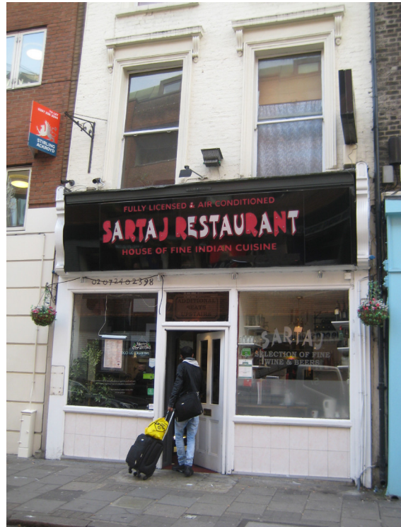
View of existing Earlham Street shopfront elevation.
