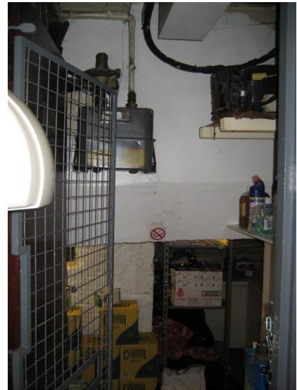
Existing Basement Vaults
