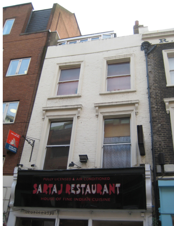
View of existing Earlham Street upper floors elevation.
