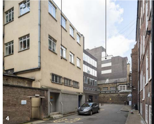
Rear of No. 19 High Holborn with No. 14-18 in foreground
