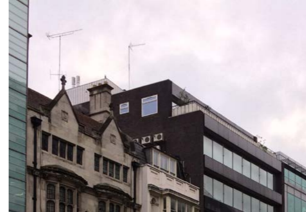
Existing internal constraints have necessitated visible external plant
