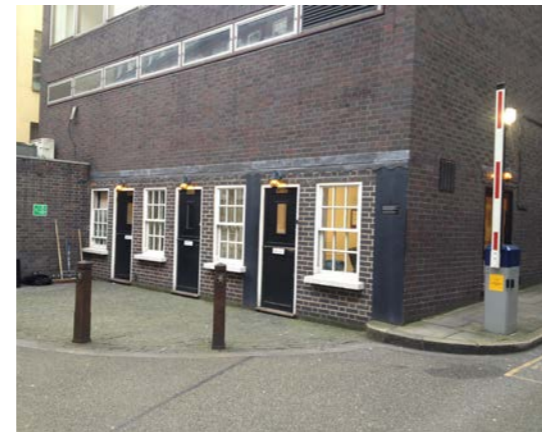
Entrance to Porters' Accommodation to rear of No. 19
