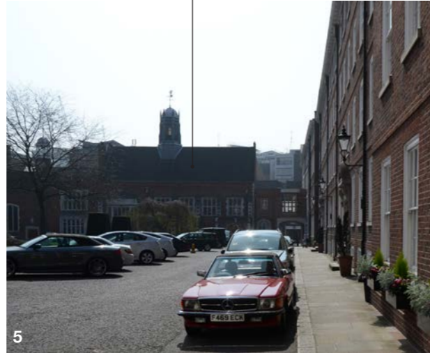
Rear of No. 19 High Holborn viewed from Gray's Inn Square between The Hall and No. 14 South Square
