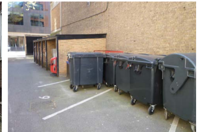
Paddock looking east. Unsatisfactory bin storage
