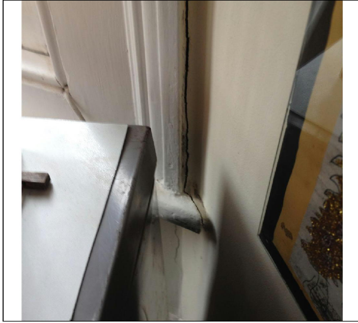
First floor front office
