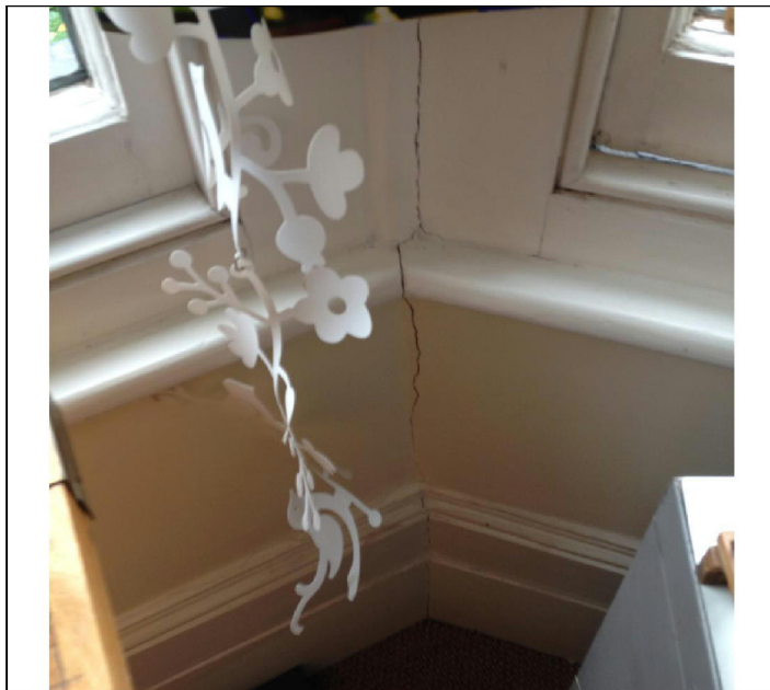
First floor front office
