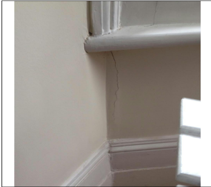
First floor front office
