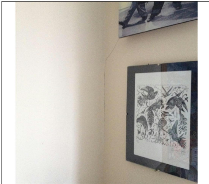
First floor front office
