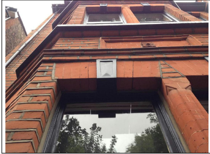
Separation to brick arch to front bay.
