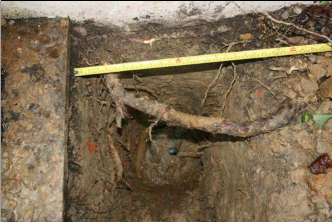
P1: Trial Pit 1 showing two roots high retaining wall at top.
