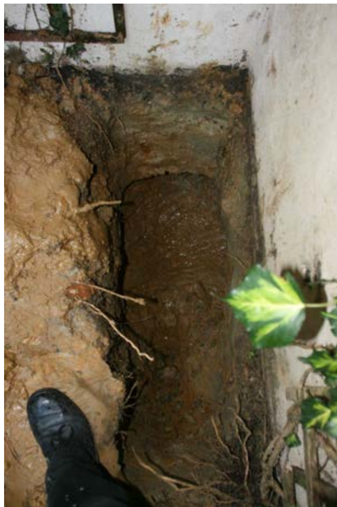
P3: Trial Pit 2 showing ivy roots near the surface.
